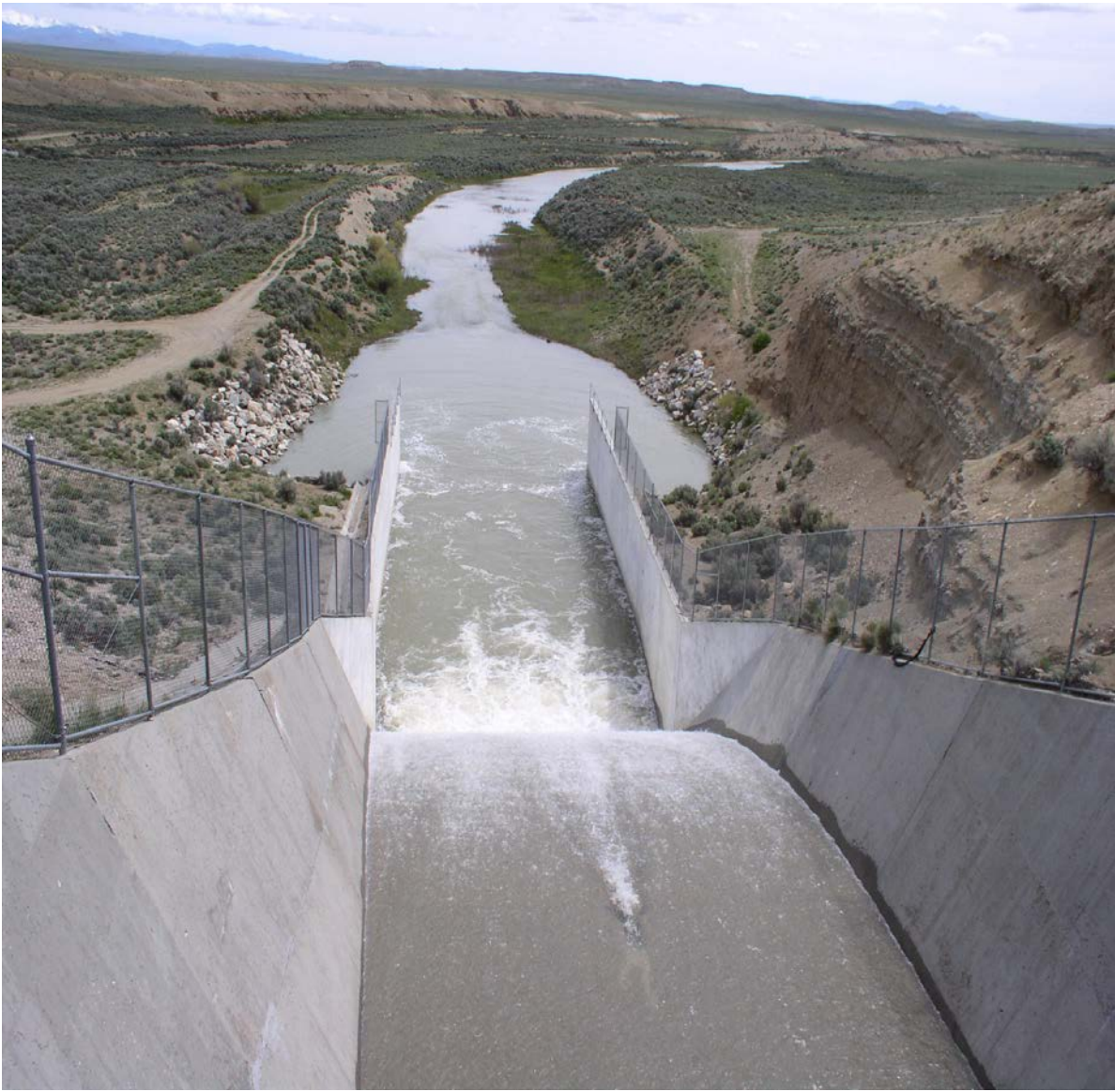
Spillway of the Big Sandy Reservoir
