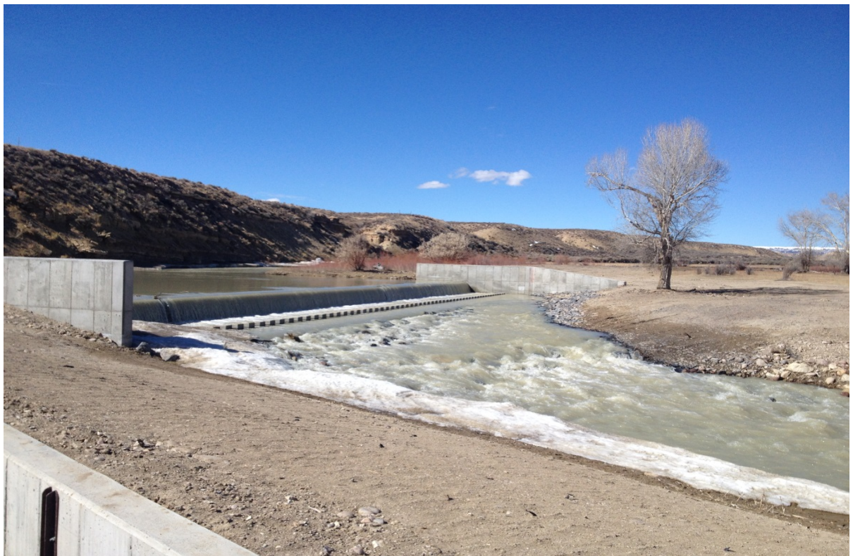
Photo 9: Peoples Canal Fish Barrier Diversion after improvements, March 2016.
