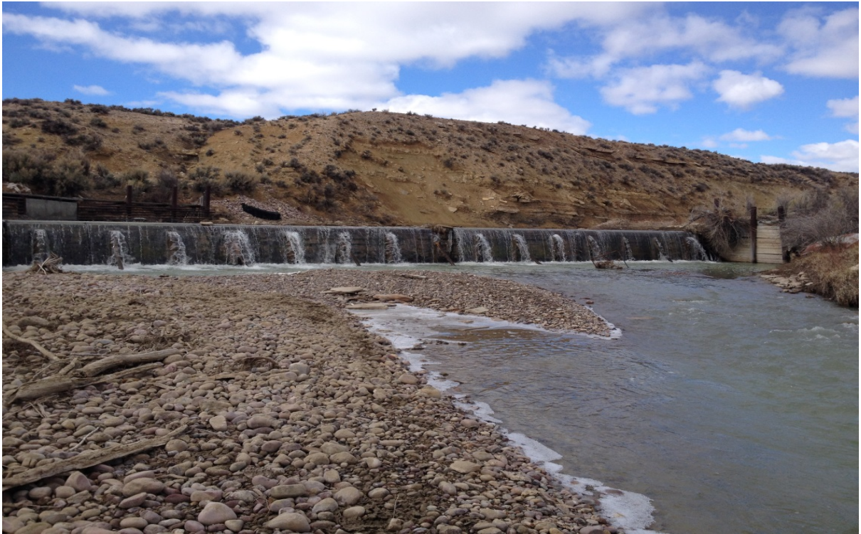
Photo 8: Peoples Canal wooden diversion prior to construction, April 2013.
