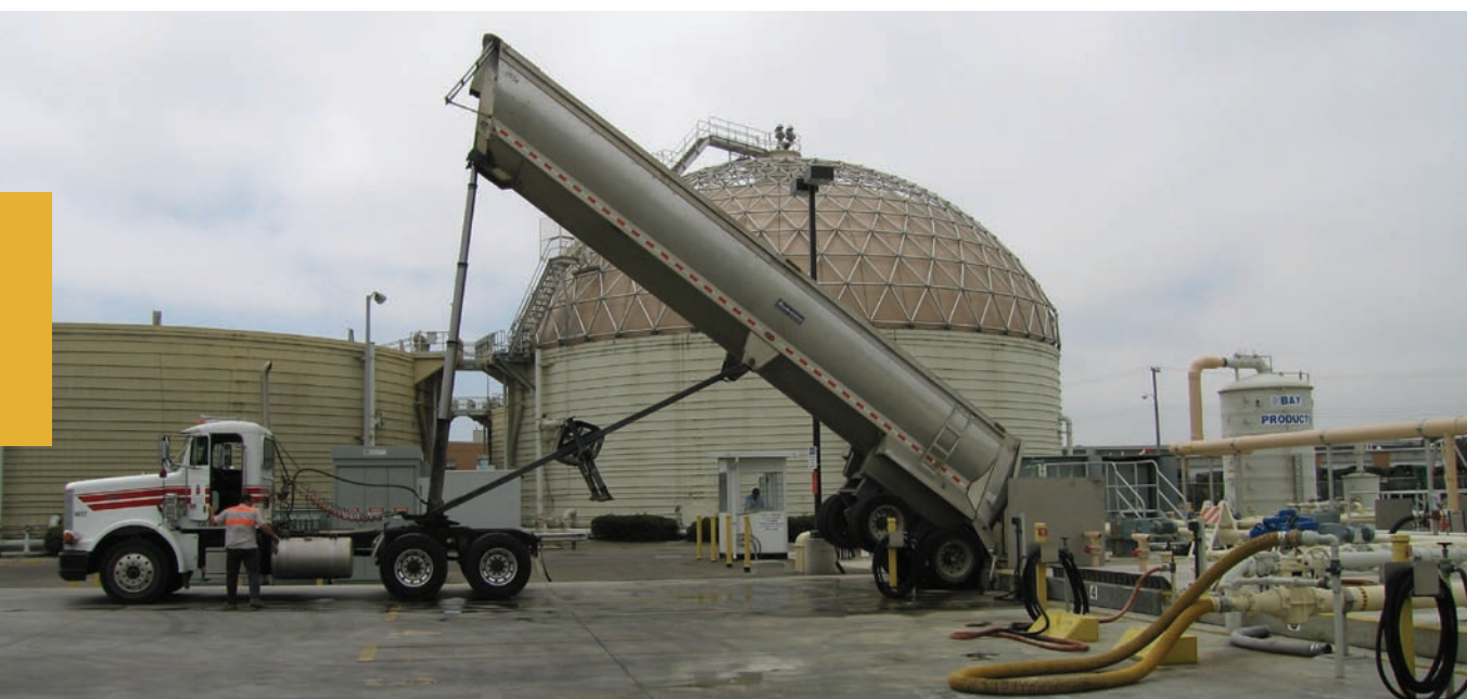
A truck off loads food waste on its way to EBMUD’s dome-shaped anaerobic digester.
