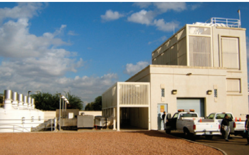
New groundwater treatment facility at the Indian Bend Wash Superfund site is the fourth and final one to be completed.
