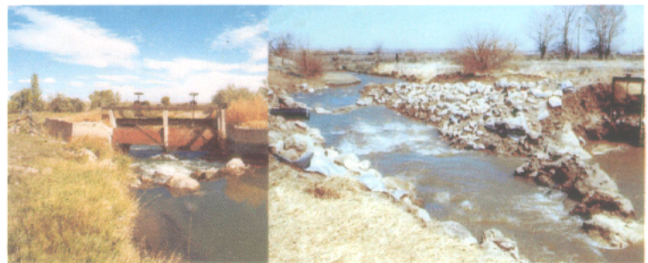
(Right) In 2001, an irrigation diversion was removed and replaced with cross vein boulder structures which provide the needed head to the irrigation diversion while providing stabilization to the stream and improved fish passage. Mill Creek, WY.
