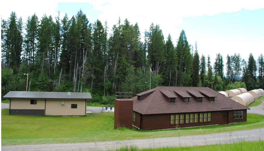
Refurbished hatchery building and new effluent treatment plant / USFWS
