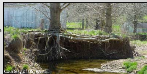
Stream with reduced riparian tree cover and an eroded bank
