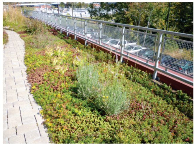
Figure 4. A green roof application.
