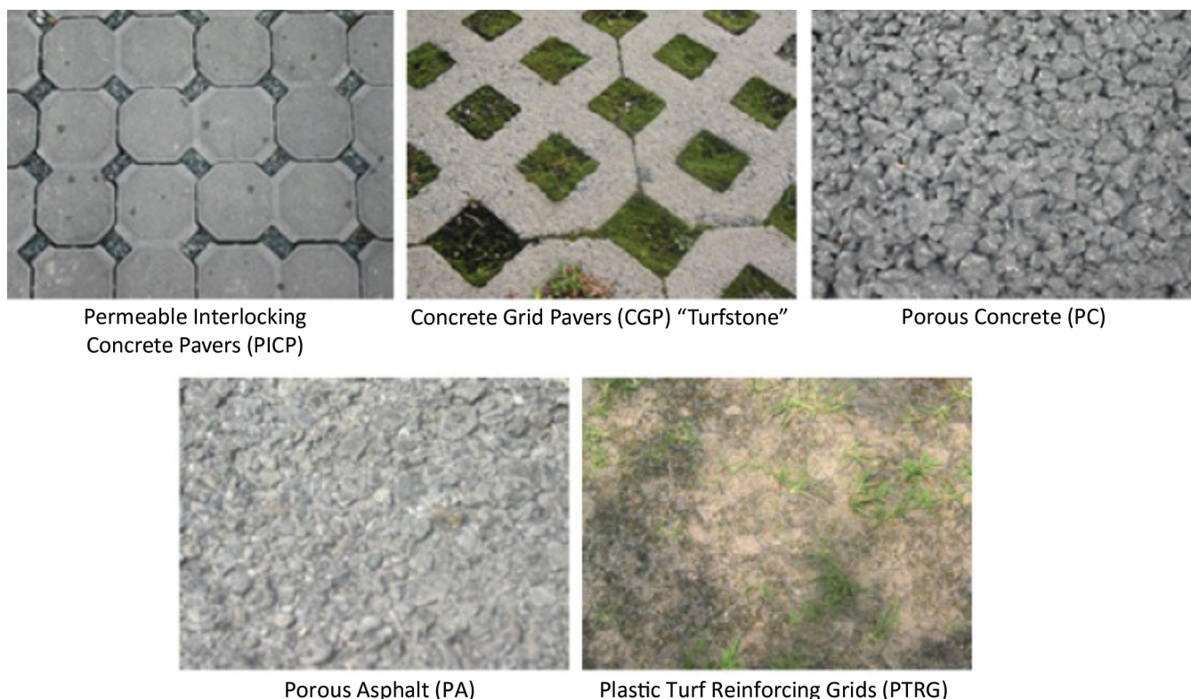
Figure 1. Examples of permeable pavement applications.
