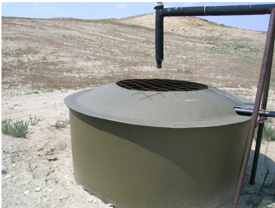
Figure 8. Dehydrator tank with a partially-covered top.
