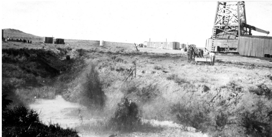
Figure 10. Discharge of oil into a dammed up gulch, Lance Creek field, Niobrara County, Wyoming, 1918 (USGS Historical Photos) (Hancock 1921).
