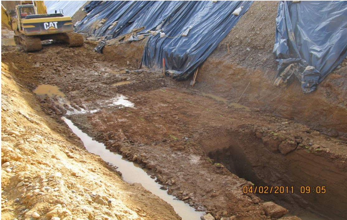
Balfour Beatty excavating pumping plant keyway trench.
