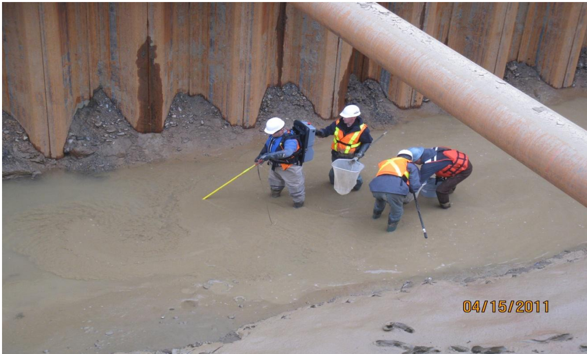
West Bay Builders subcontractor FishBio performing fish rescue in the siphon.
