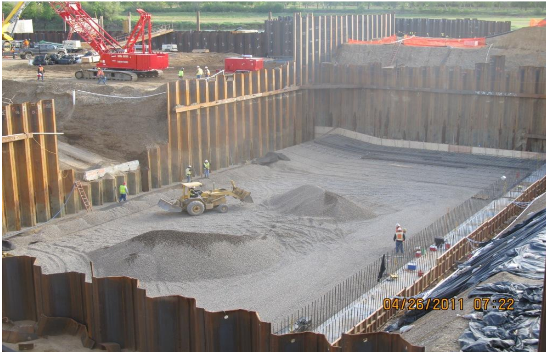
Balfour Beatty placing crushed rock over geotextile for pumping plant sub-base.
