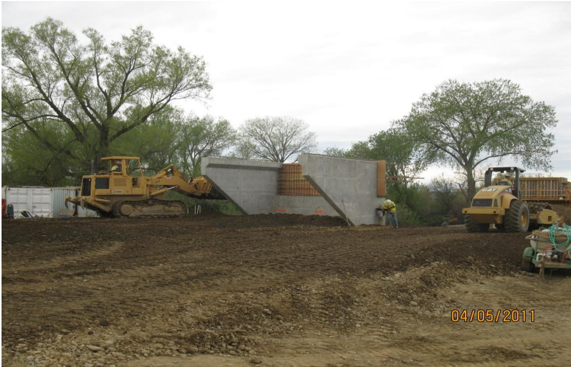
West Bay Builder's subcontractor Meyers backfilling east bridge abutment.
