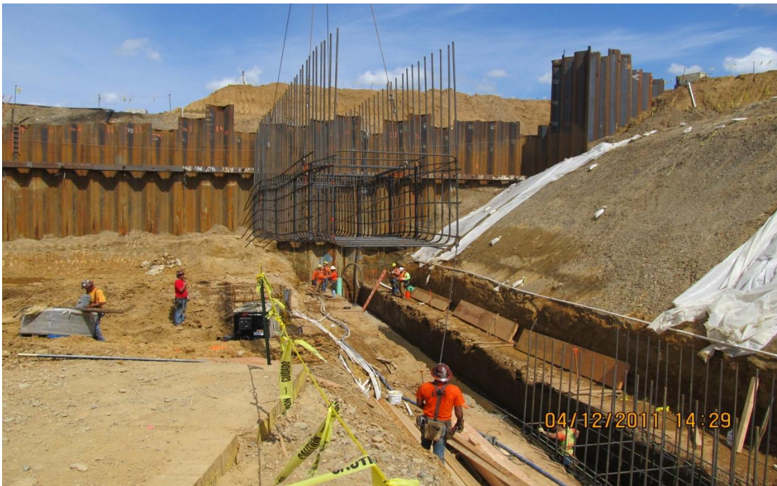
Balfour Beatty crane hoisting reinforcing cages into pumping plant for Keyway.
