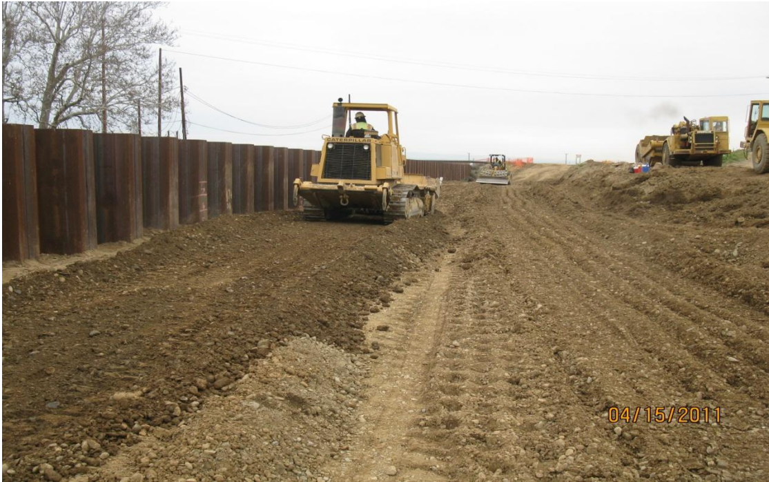
West Bay subcontractor Meyers backfilling south side of downstream canal.
