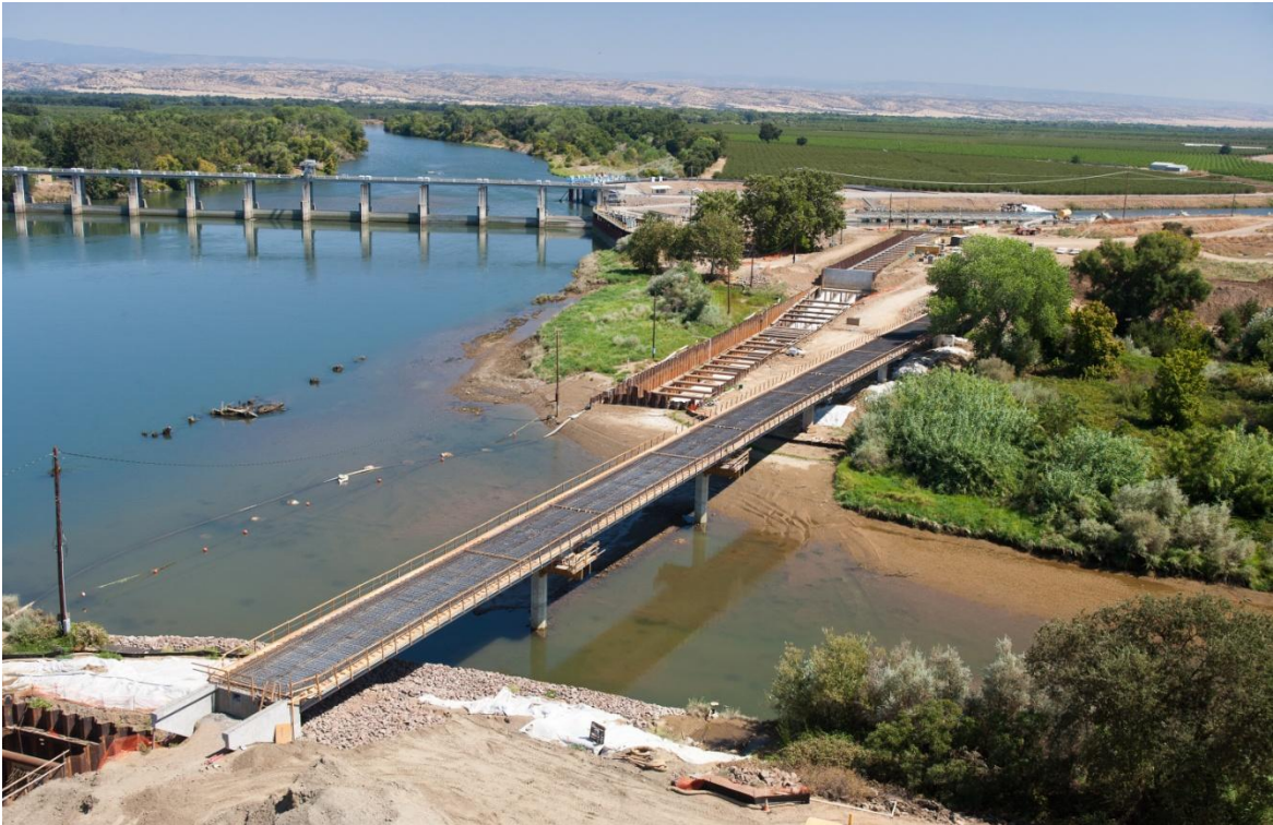
Aerial view of bridge.
