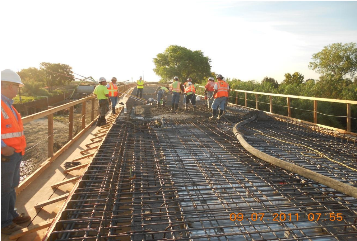
West Bay Builders bridge deck concrete placement.
