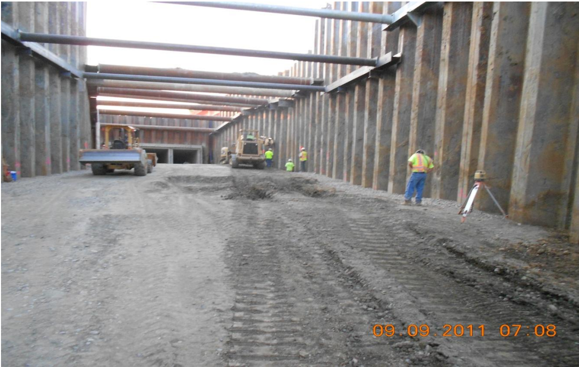
West Bay Builders siphon inlet structure sub grade preparation.
