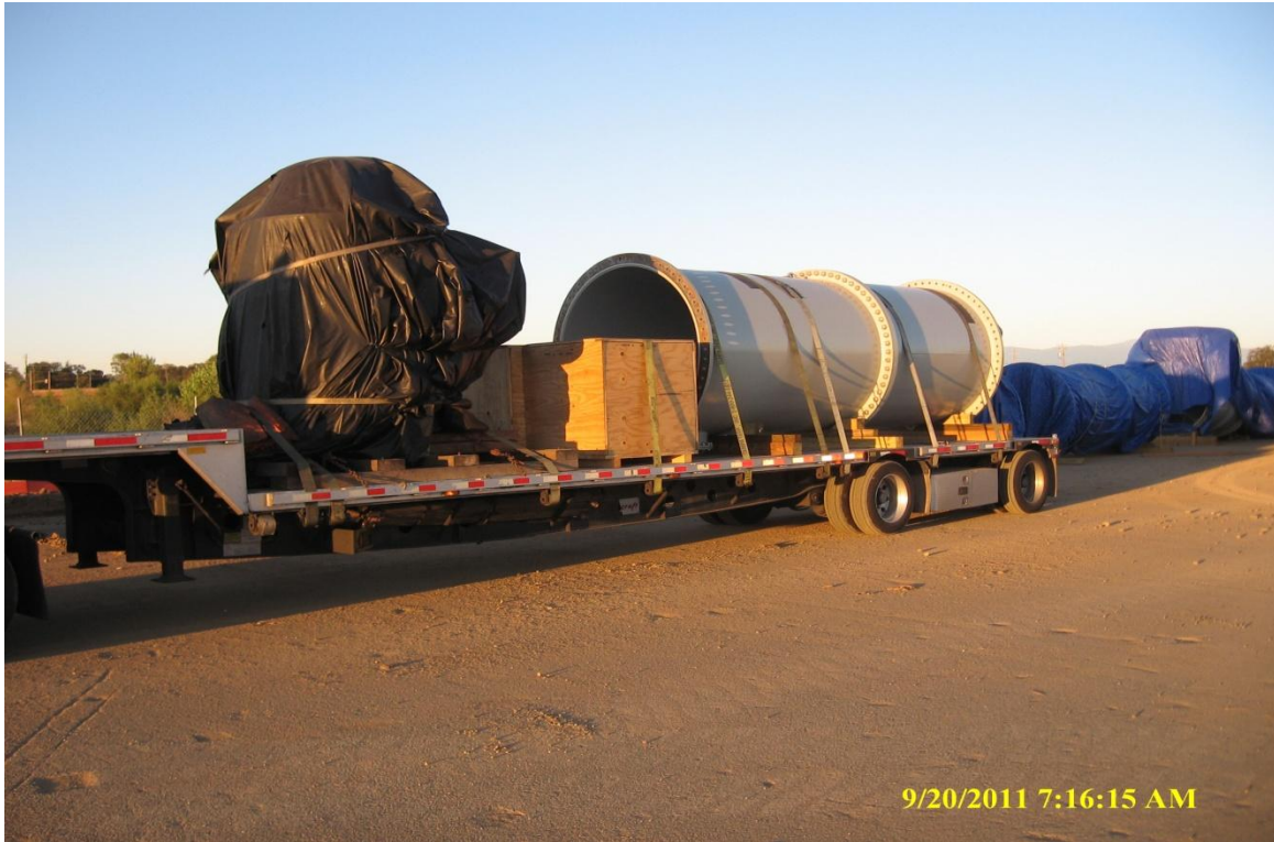
Balfour Beatty delivery and off load of pumps and motors.
