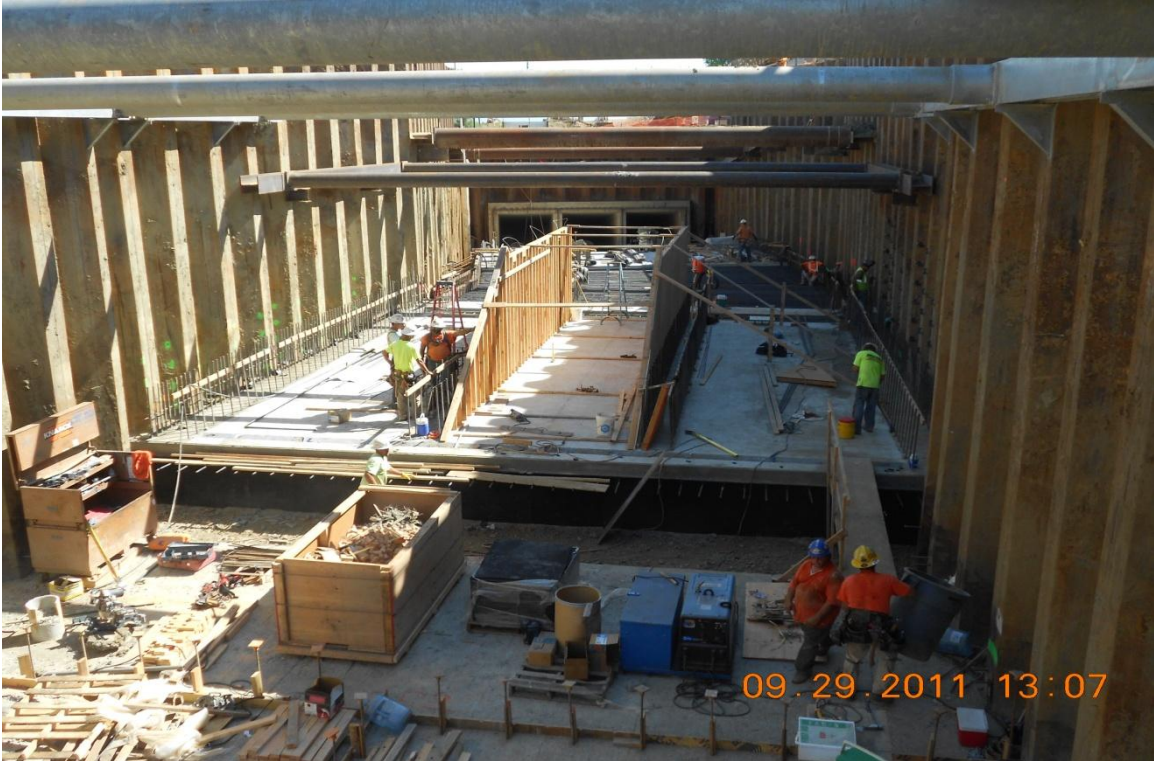
West Bay Builders working on inlet structure wall forms.
