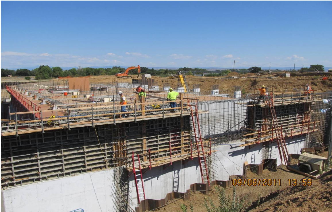
Balfour Beatty pumping plant wall placements.
