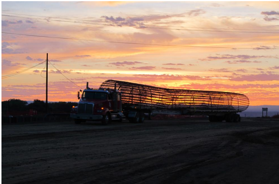
West Bay Builders Delivering Reinforcement Cage for Bridge Piers
