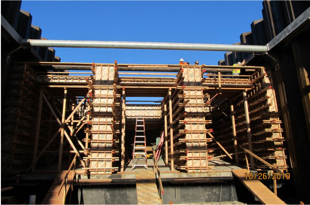
Siphon Outlet Structure
