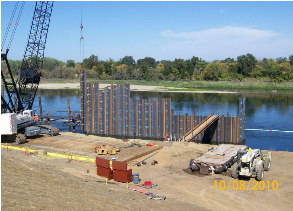
Installing Cofferdam Sheet Piling for Fish Screen Bay 14
