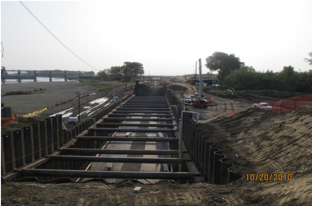
Siphon Barrel Structure
