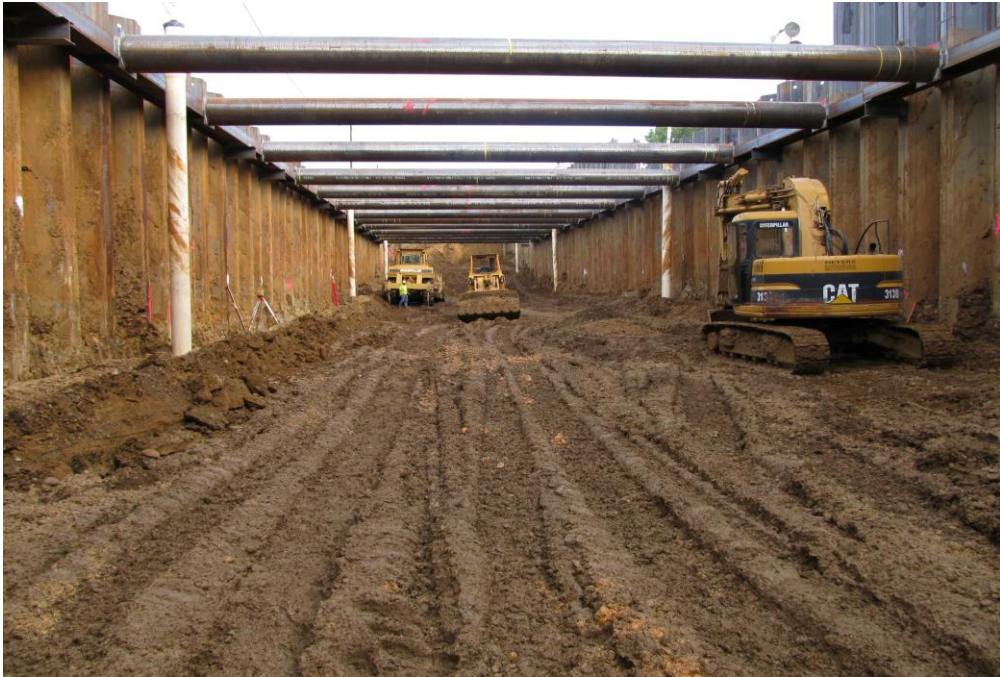
West Bay Subcontractor Excavating Siphon Structure
