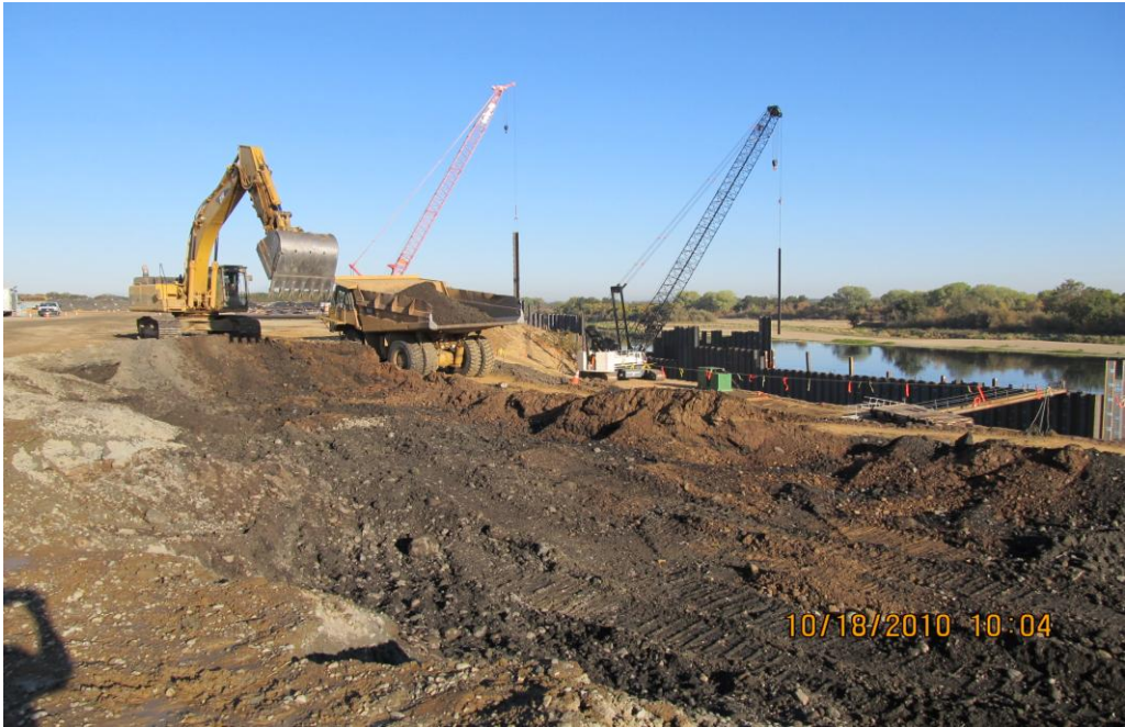
Pacific States Construction Excavating from Pumping Plant and Fish Screen
