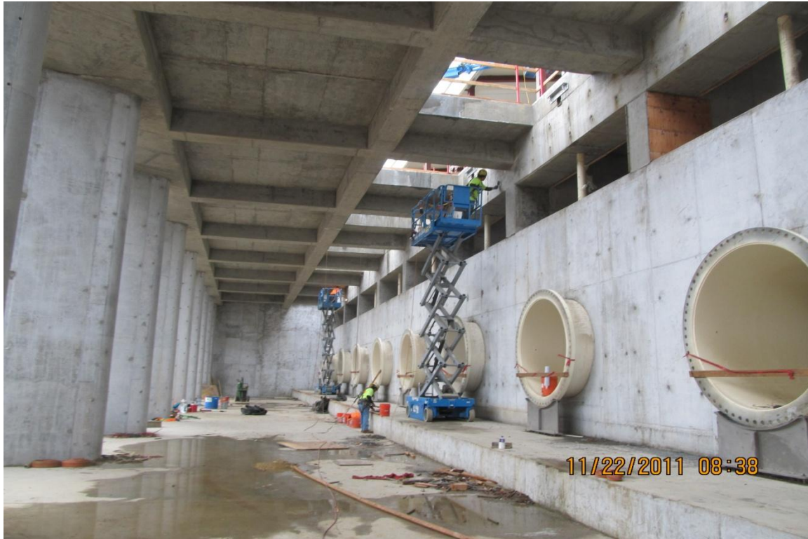
Balfour Beatty labor crew removing formwork from discharge wall of afterbay.
