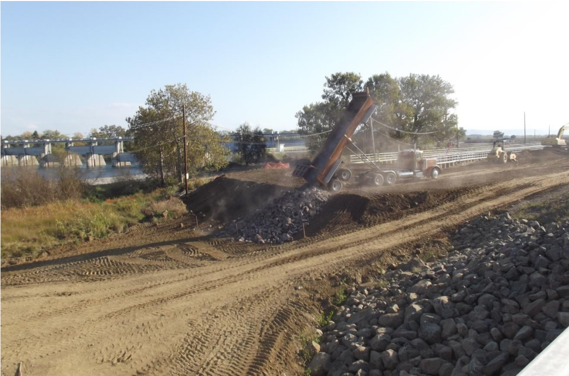
West Bay Builder subcontractor Meyers Earthwork placing rip rap.
