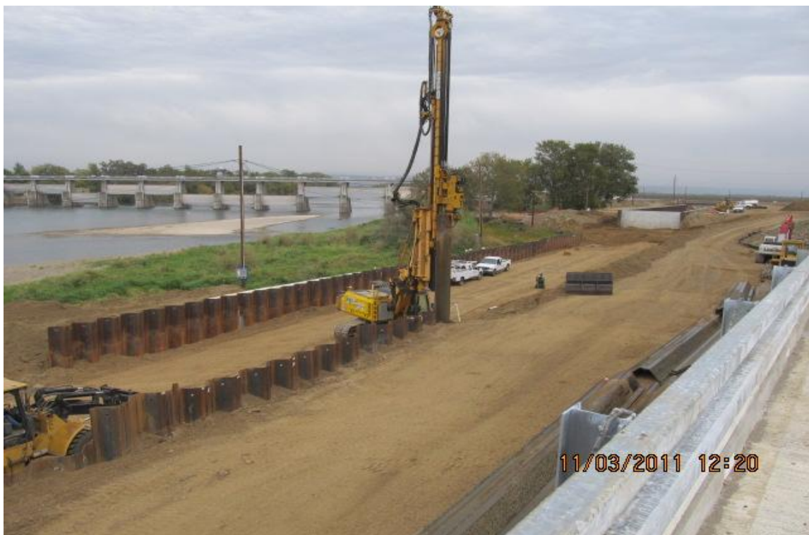
West Bay Builders subcontractor Hughes Construction removing temporary sheet pile.
