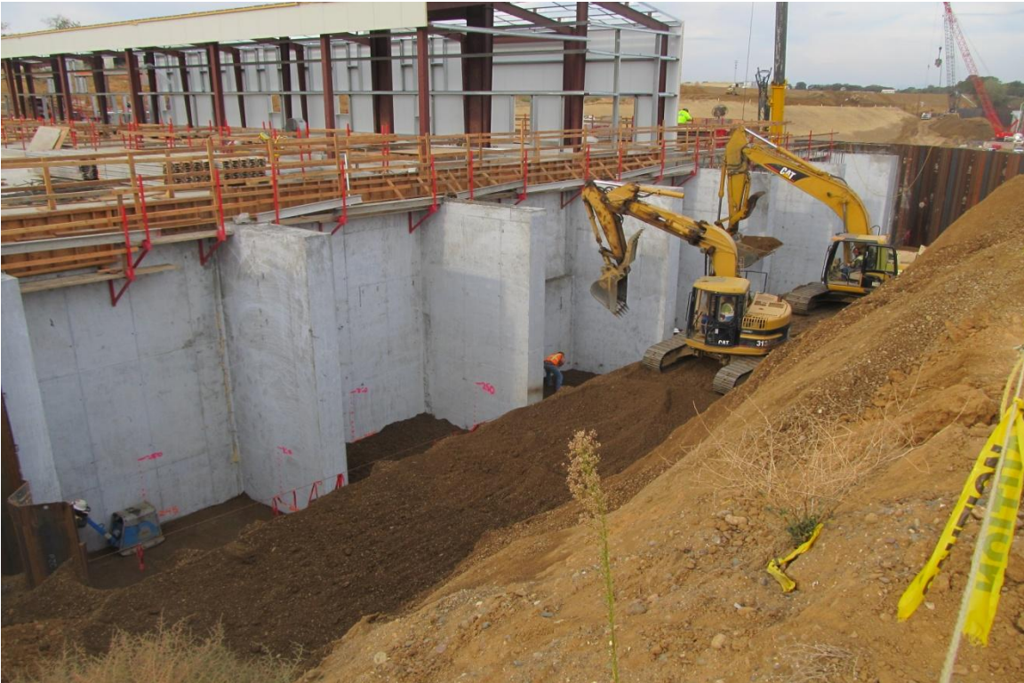
Balfour Beatty subcontractor Meyers Earthwork back filling at pumping plant.
