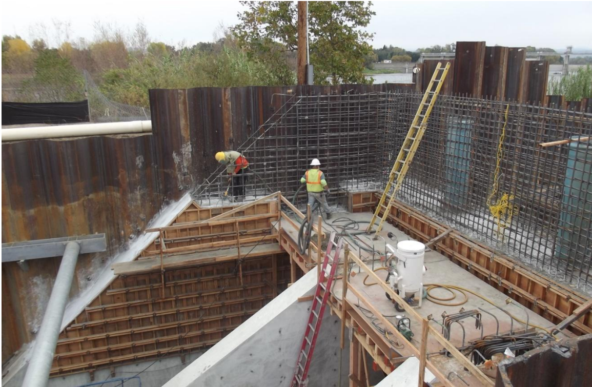
West Bay Builders labor crew sand blasting inlet structure.
