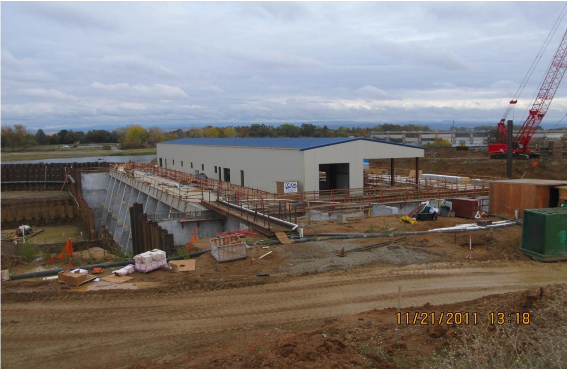
Balfour Beatty Pumping Plant Control Building roof and siding erected.
