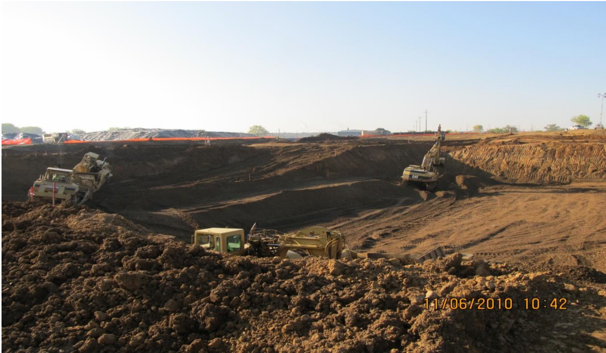
Excavation for Red Bluff Pumping Plant
