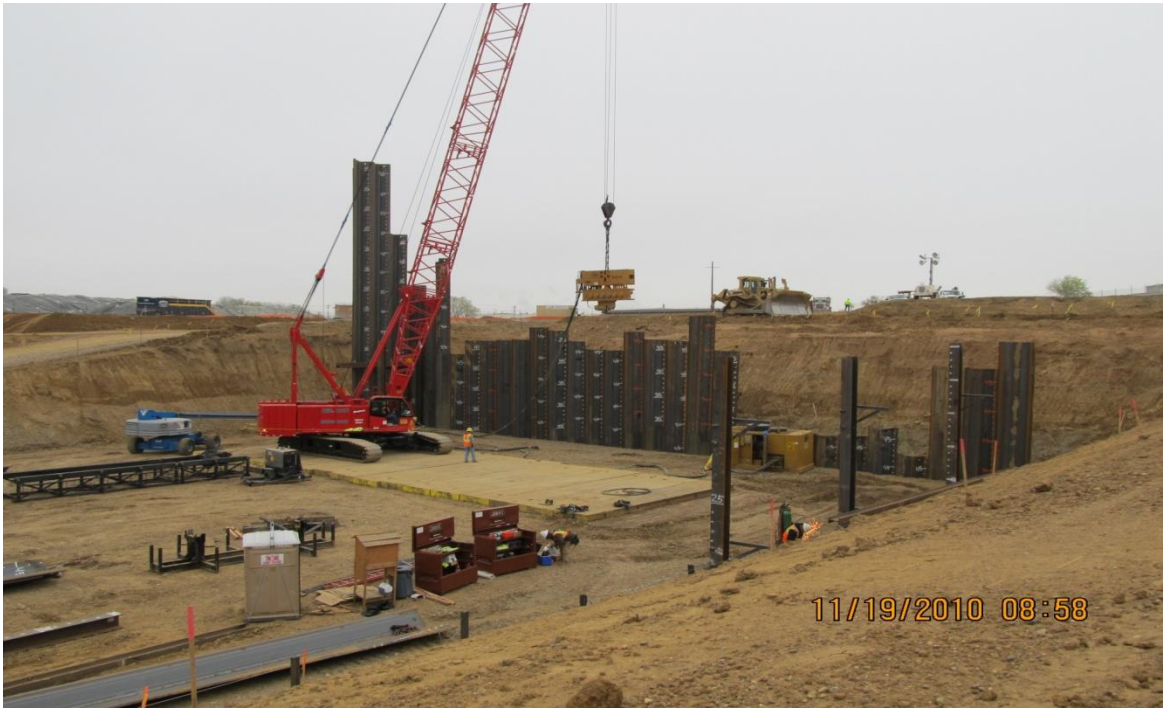
Installation of Excavation Support and Protection Sheet Piling
