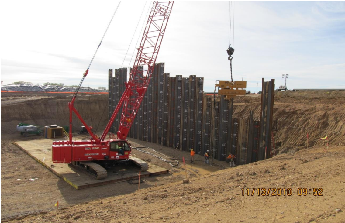
Driving Pumping Plant Sheet Piling for South Wall
