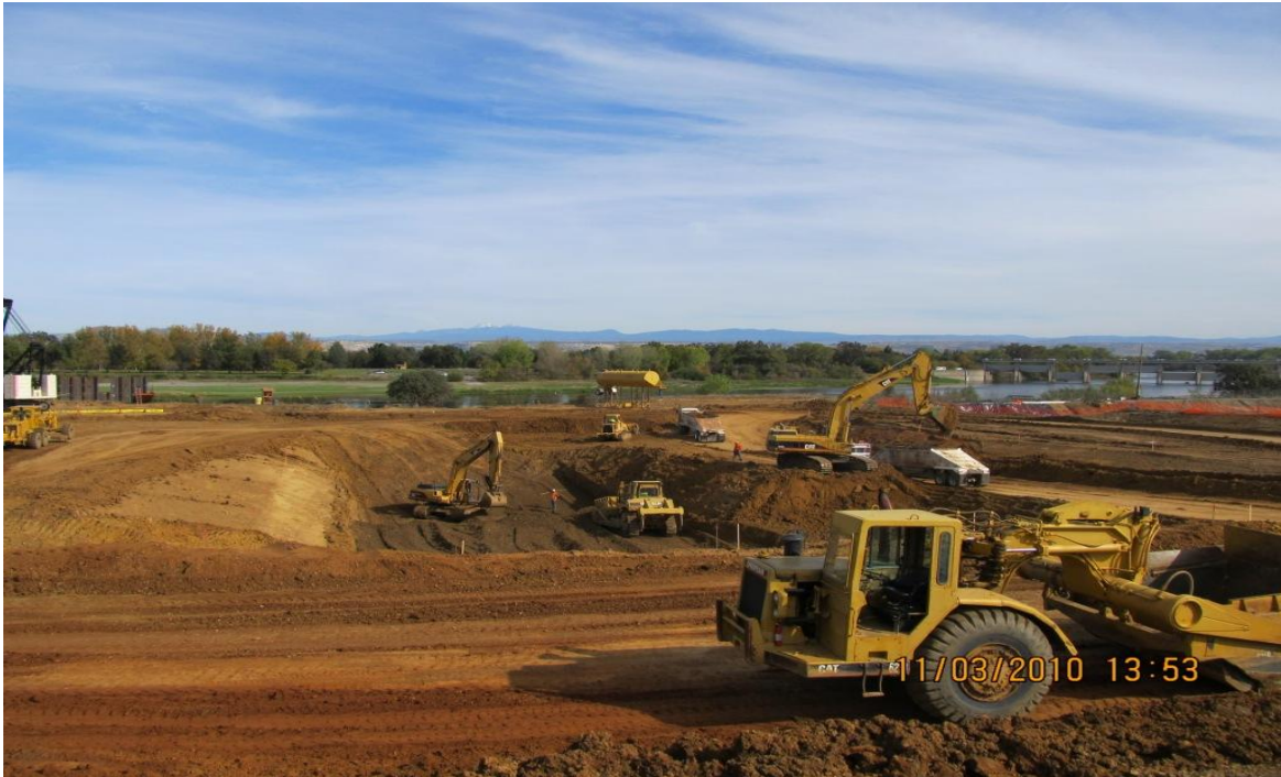
Balfour Beatty Infrastructure Subcontractor Meyers Excavating for the Future Pump Plant
