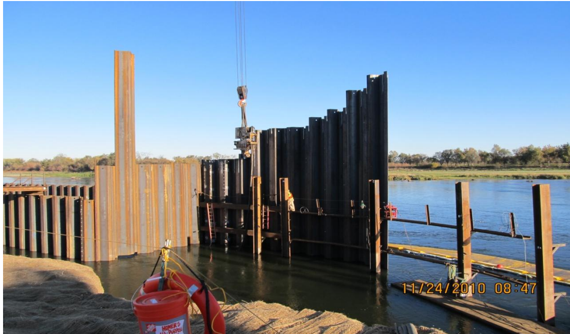
Red Bluff Downstream (East End) Section Fish Screen Sheet Piling Installation
