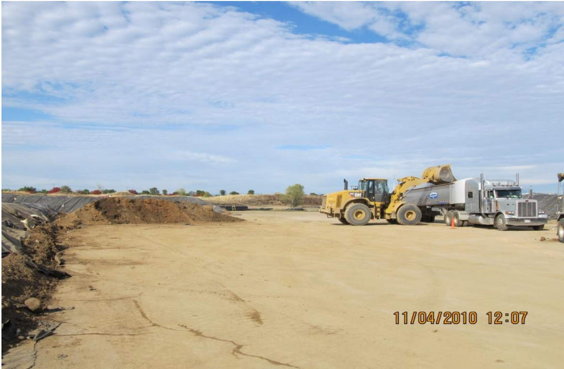
Subcontractor Pacific States Loading and Hauling Soil Material to the Landfill
