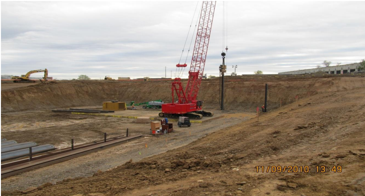
Placing H (pin) Piles for Pumping Plant Sheet Piling Guides
