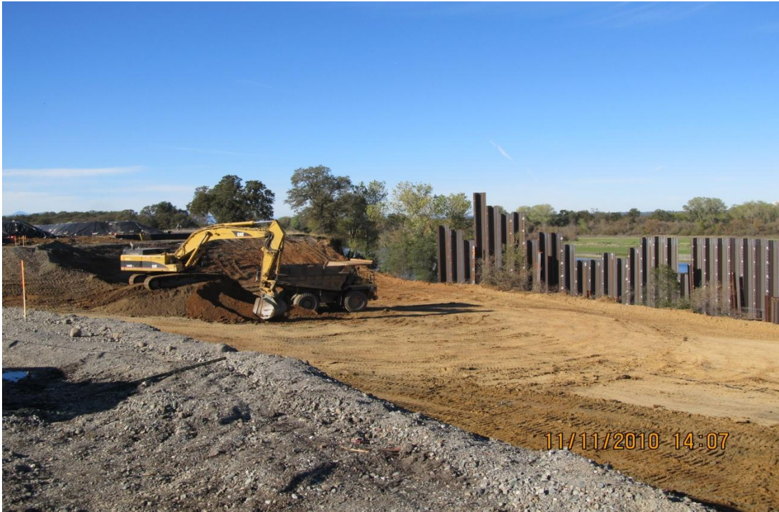
Excavation of Material from Forebay at Upstream End
