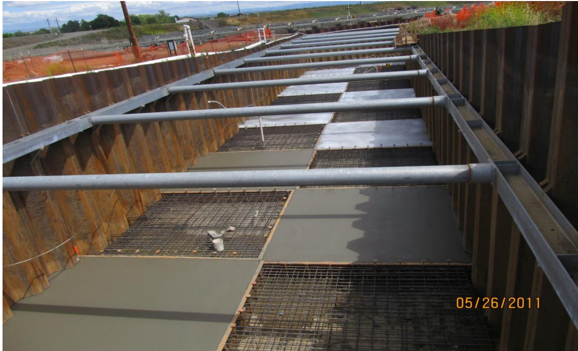
West Bay Builders downstream structural concrete placed in interval bays.
