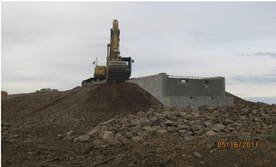
West Bay Builders subcontractor Meyers working on east bank slope protection.
