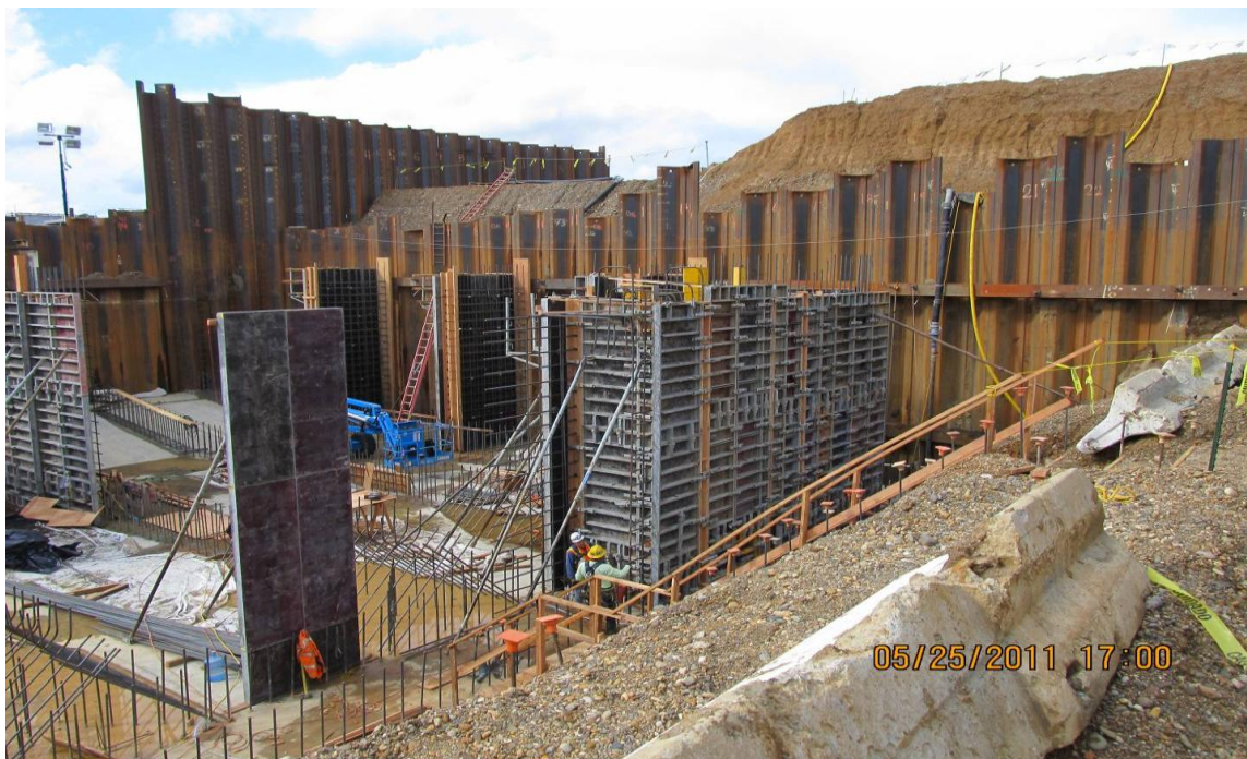
Balfour Beatty pumping plant back wall formwork.
