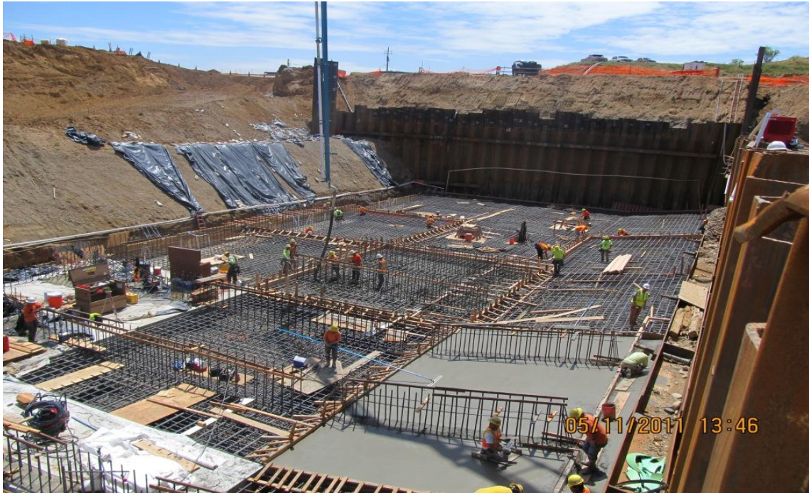
Balfour Beatty placing concrete for pumping plant sump slab.
