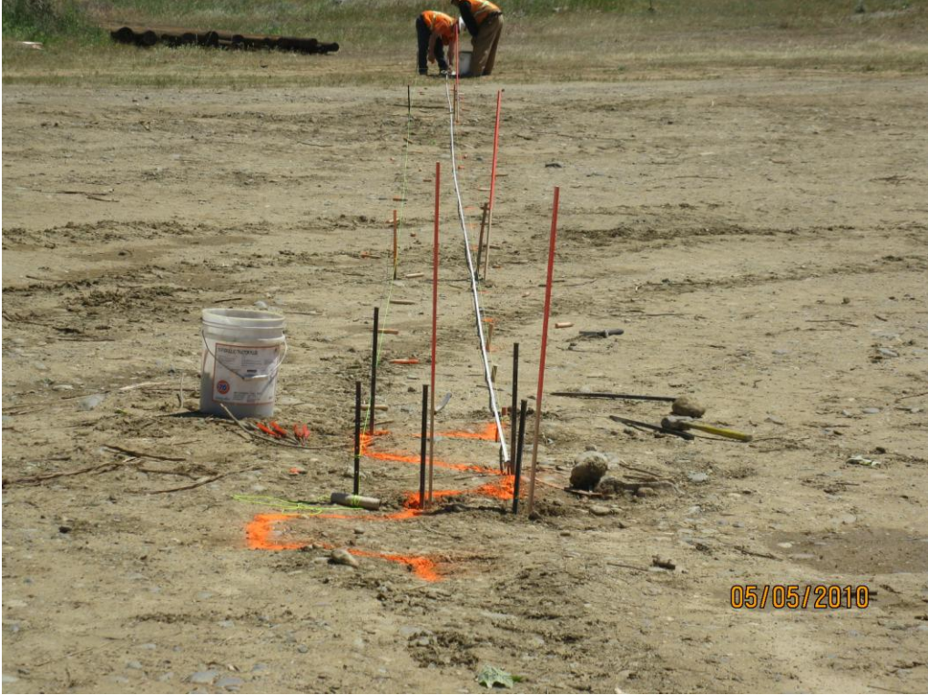
Laying out the Sheet Pile locations.
