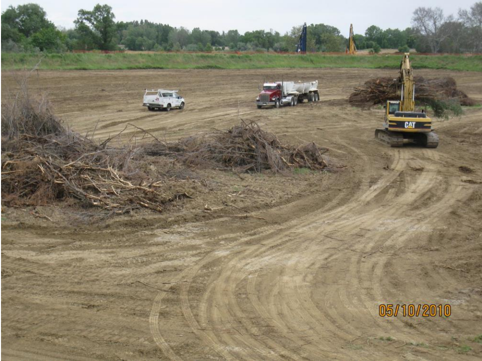
Clearing and Grubbing the sediment ponds.
