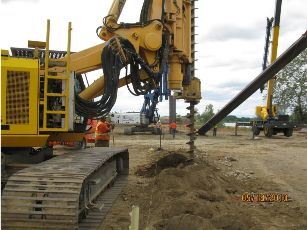
Pre-drilling before driving the sheet piles.
