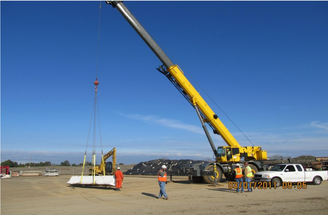
Balfour Beatty performs a load test on a hydraulic crane.
