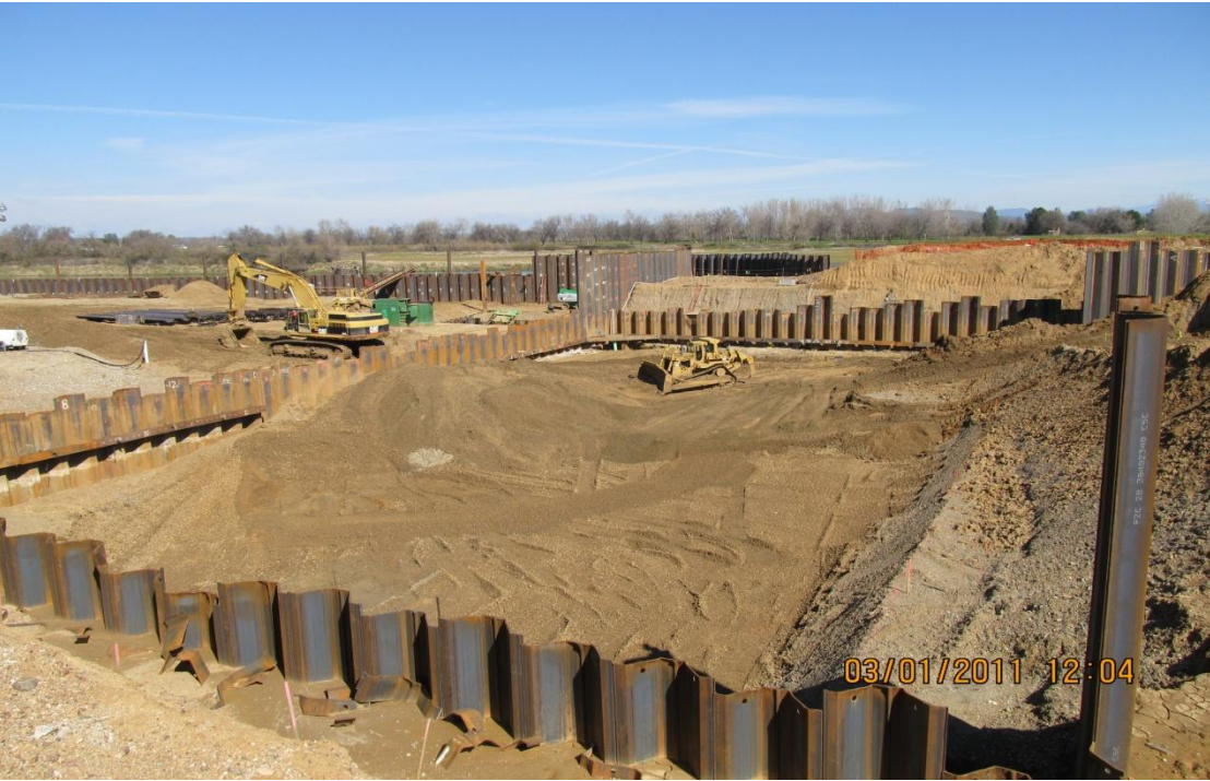
Balfour Beatty's subcontractor Meyers excavates in the pumping plant.
