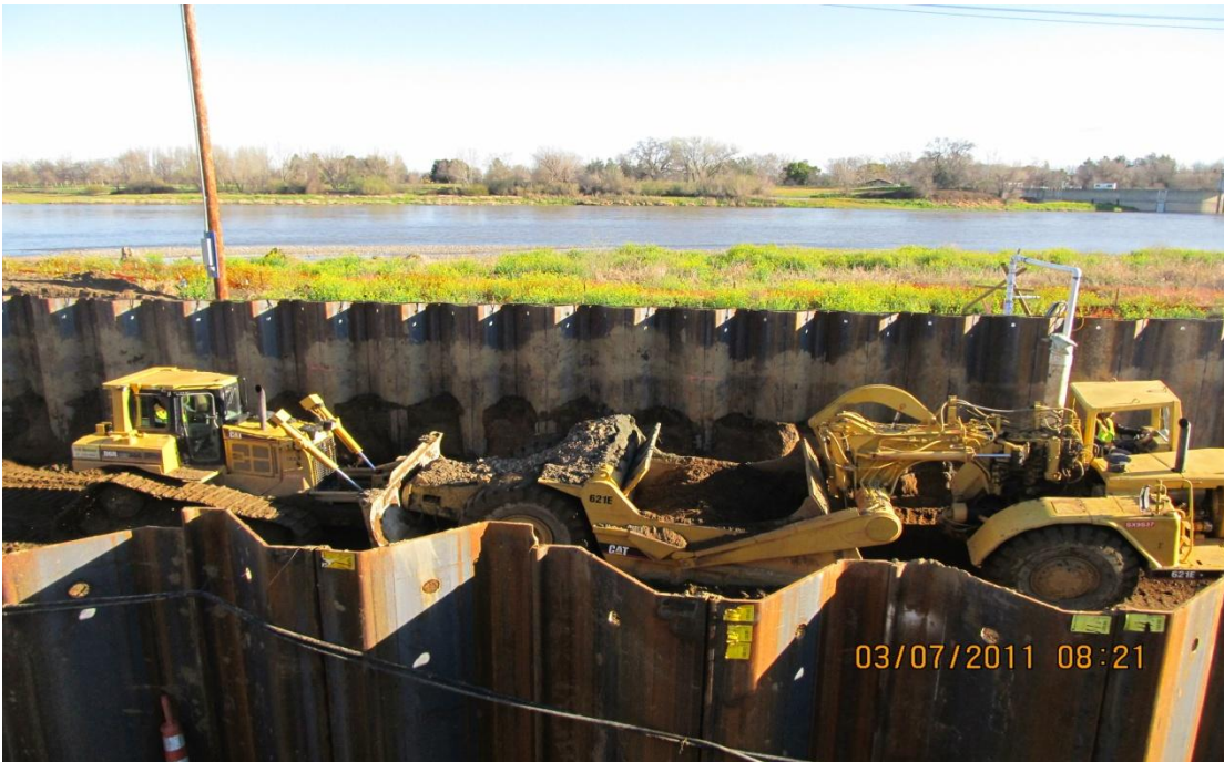
West Bay subcontractor Meyers excavating the first lift of Phase 2 Siphon.
