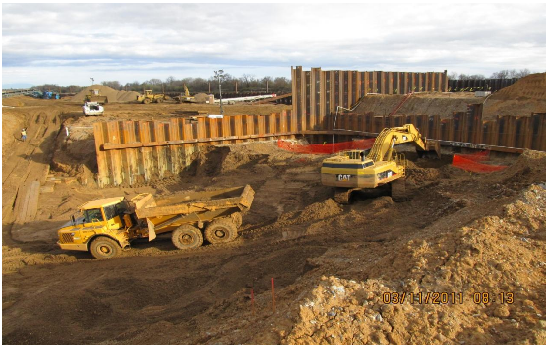
Balfour Beatty subcontractor Meyers excavating the pumping plant.
