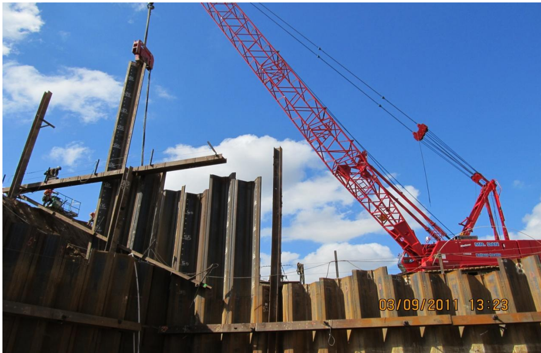
Balfour Beatty crane drives sheet pile for upper forebay wall.
