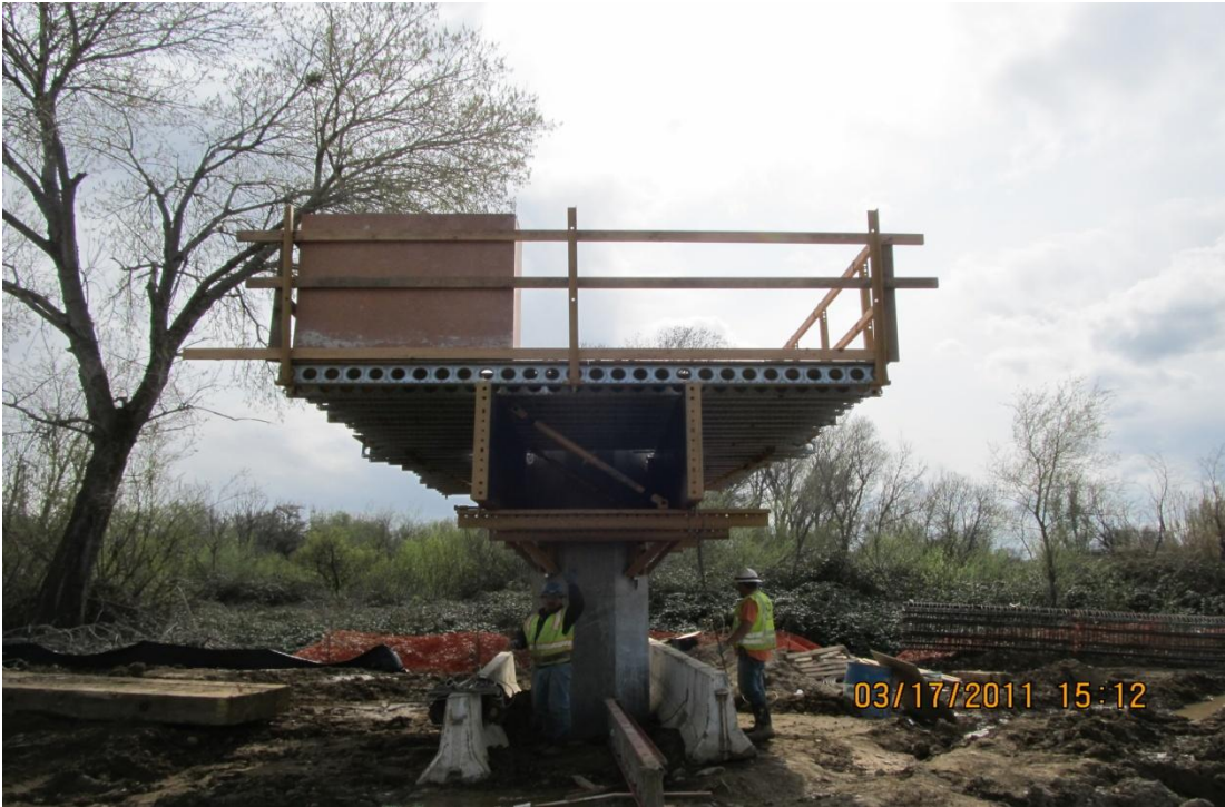
West Bay Builders installs the EFCO forms for Column #5.
