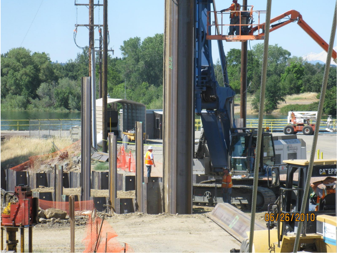
Pile driving through dike #2.
