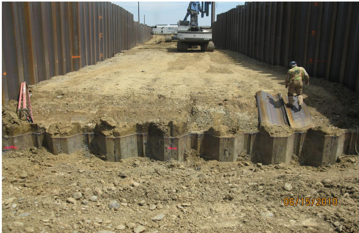
Looking down the new canal section east of Red Bank Creek.
