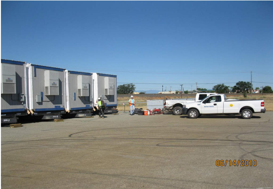
Balfour Beatty mobilizing onto the job site.
