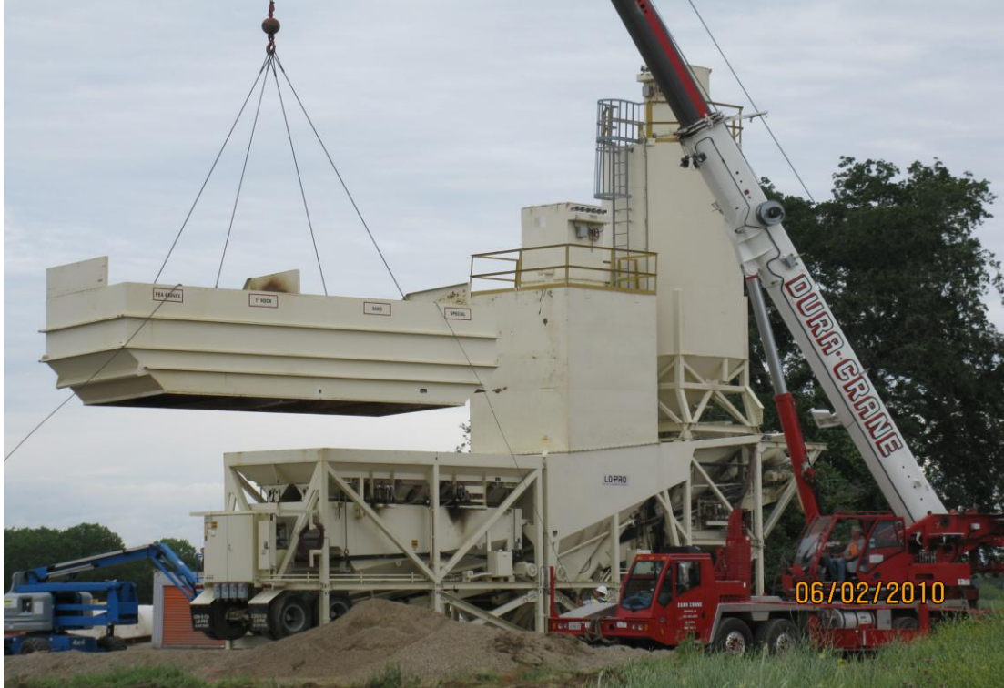
Assembling portable concrete batch plant for onsite concrete production.
