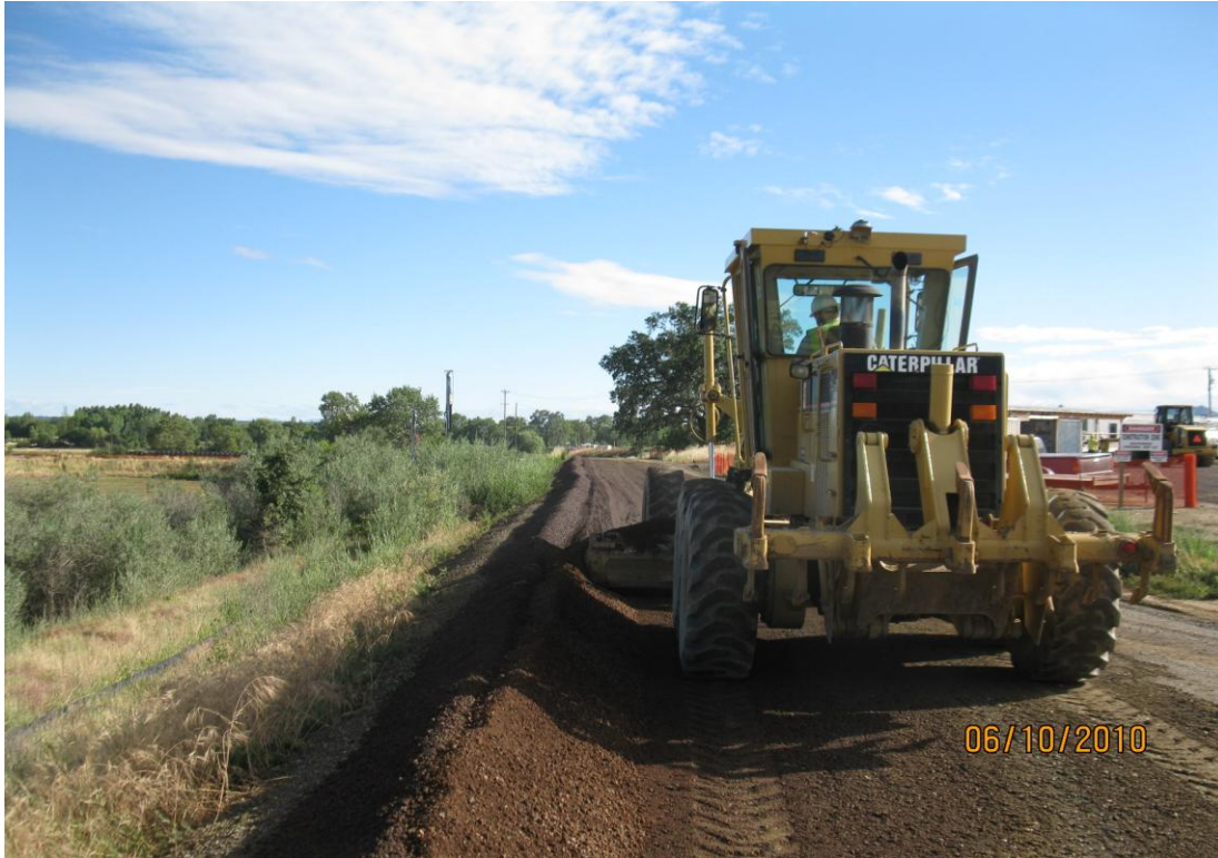
Meyers Earthwork building a service road east of sediment pond #1.
