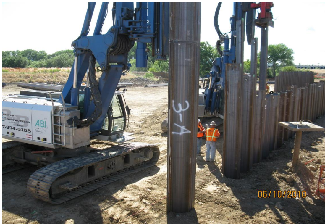
Driving sheet piles with both vibratory hammer and diesel impact hammer.
