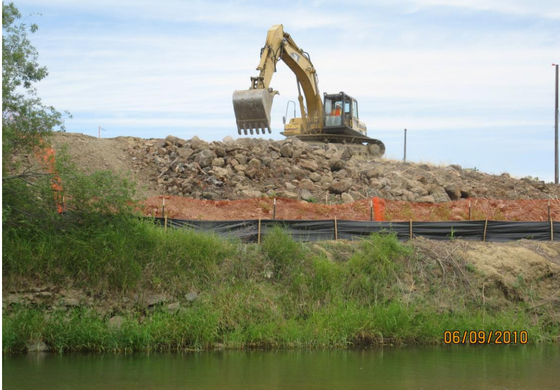
Meyers Earthwork building an access ramp.
