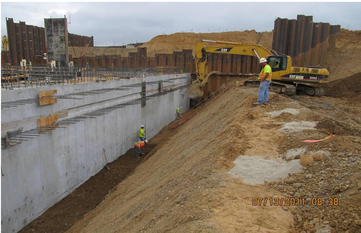
Balfour Beatty backfill operation behind discharge wall in forebay.
