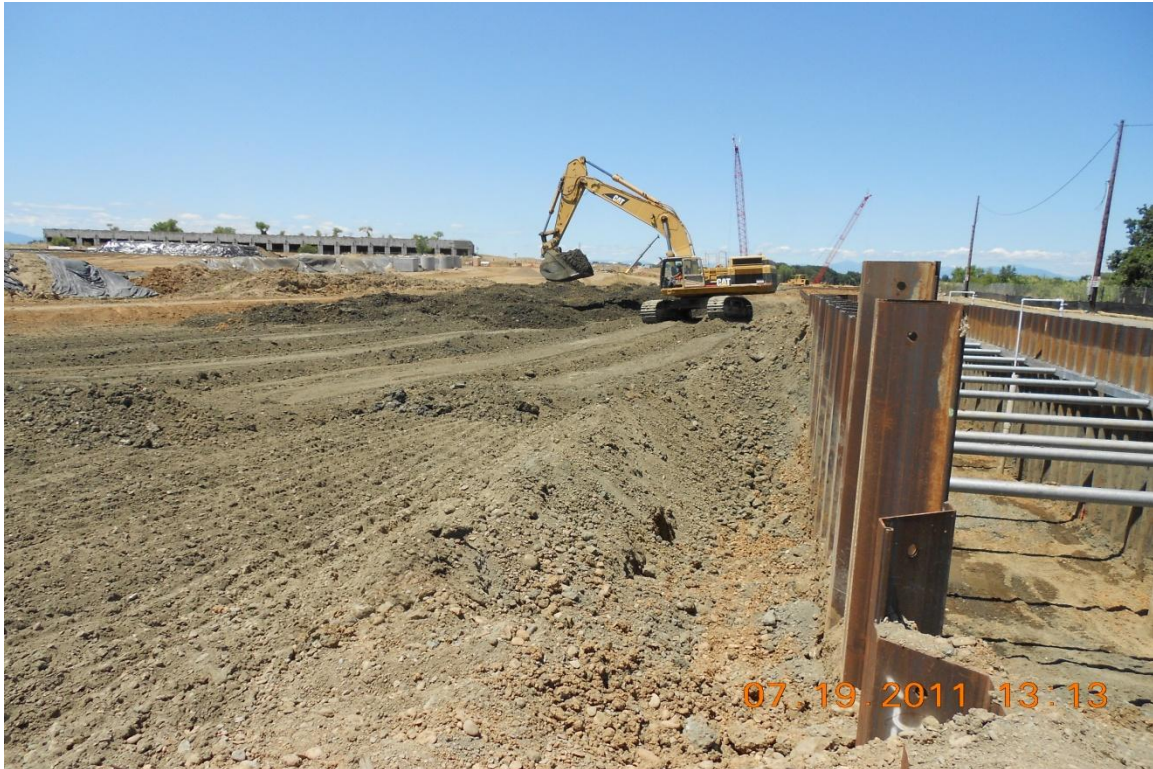
West Bay Builders' excavator digging at Upstream Canal.
