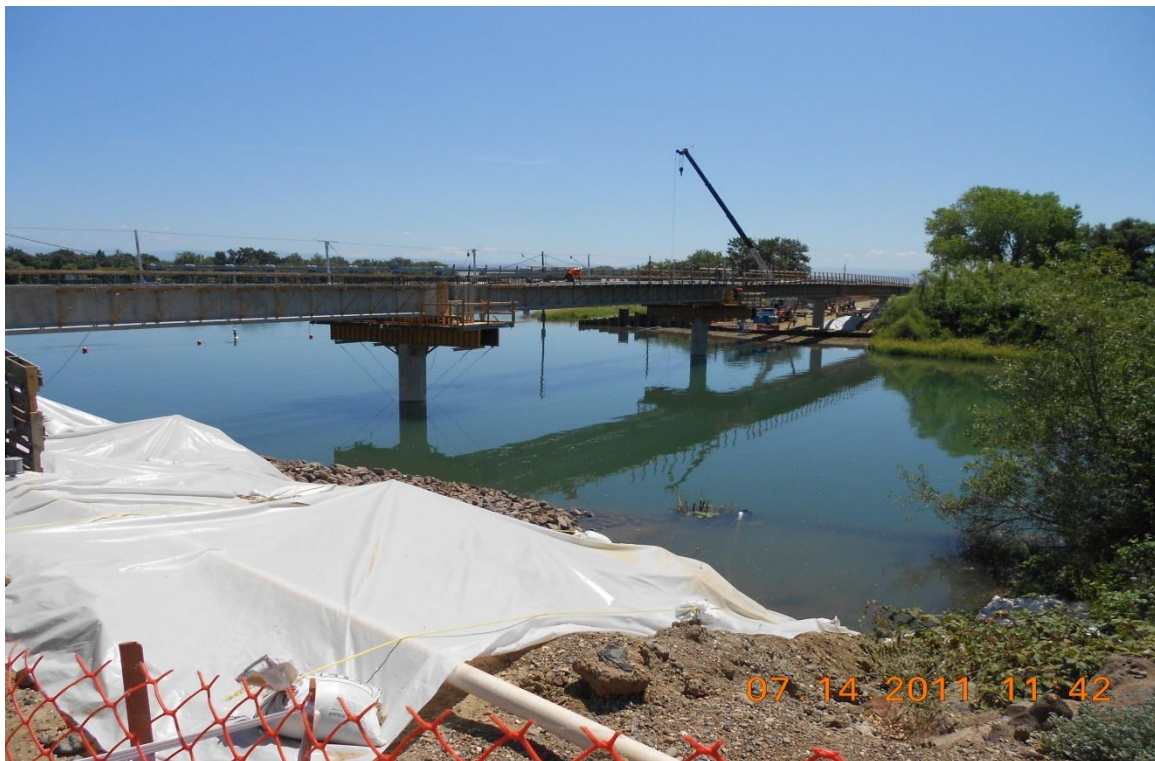
Bridge constructed by West Bay Builders crossing Red Bank Creek
