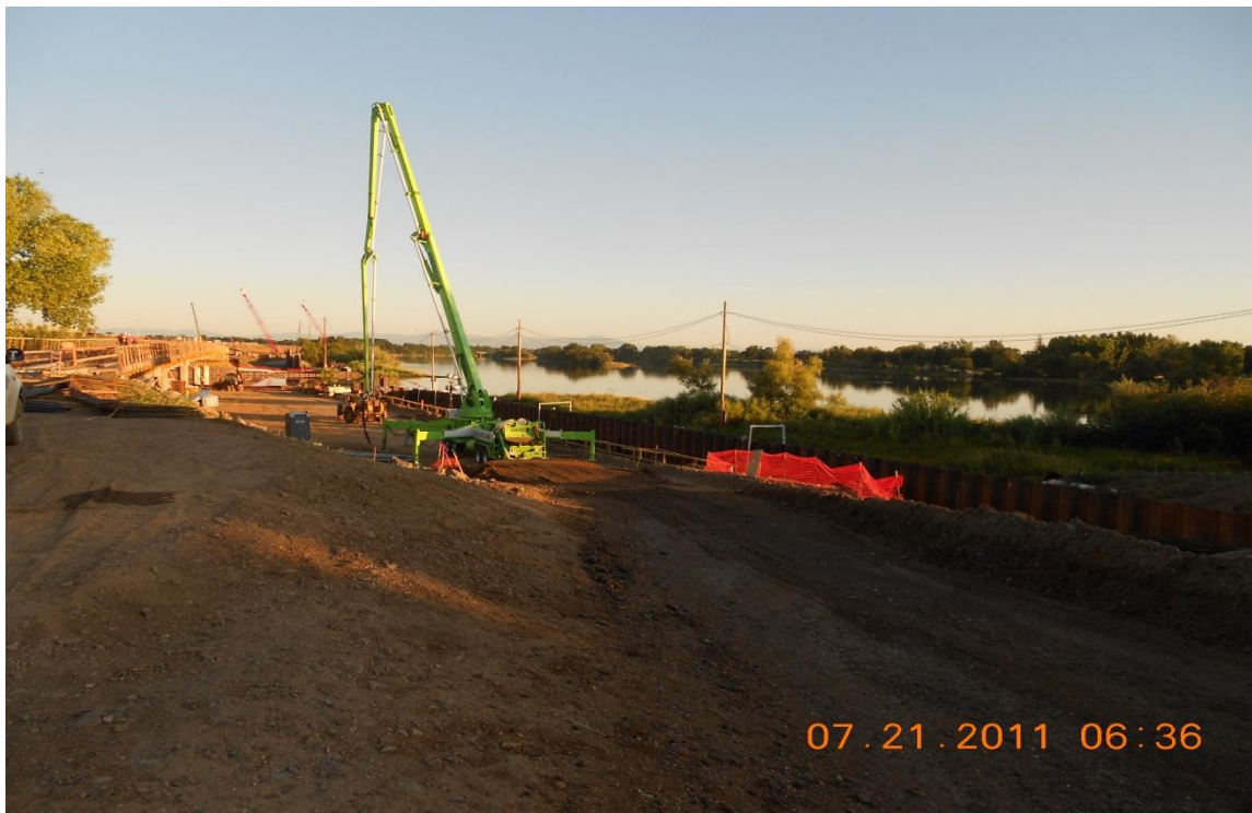
West Bay Builders concrete pump truck setting up for siphon placement.
