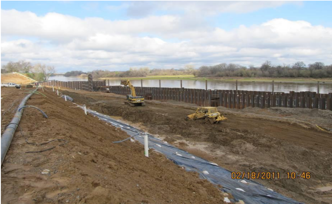
Balfour Beatty forebay dewatering and excavation.
