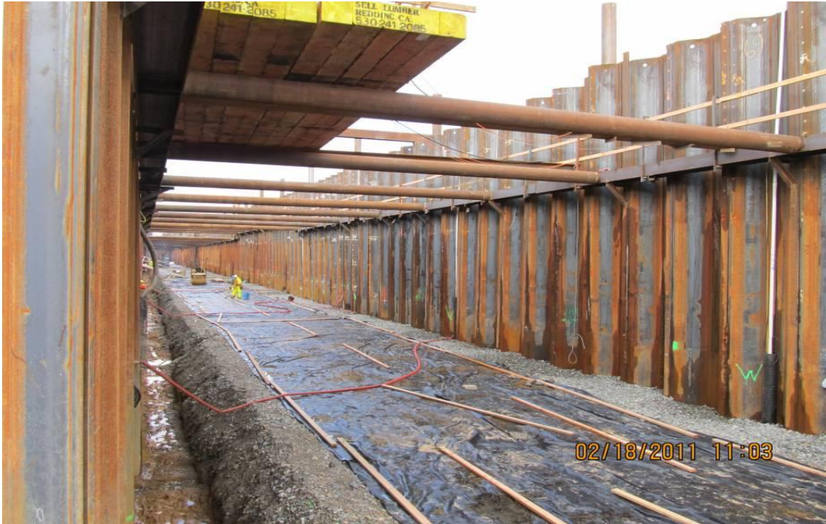
Balfour Beatty placing geotextile inside fish screen cofferdam.
