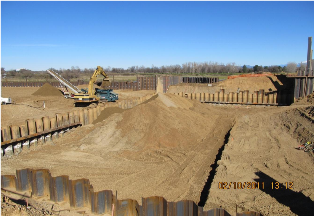
Balfour Beatty's subcontractor Meyers removing material from the pumping plant.
