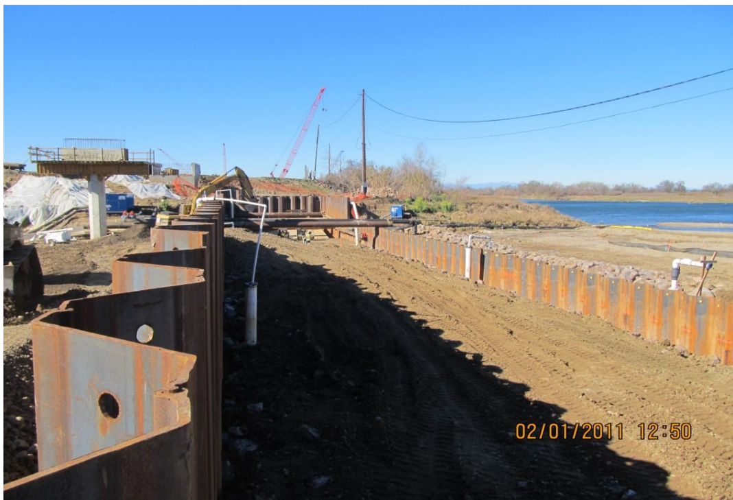
West Bay Builders grade control structure over siphon barrel structure.
