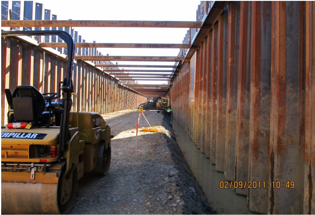
Balfour Beatty's vibratory roller inside Cofferdam Cell #2.
