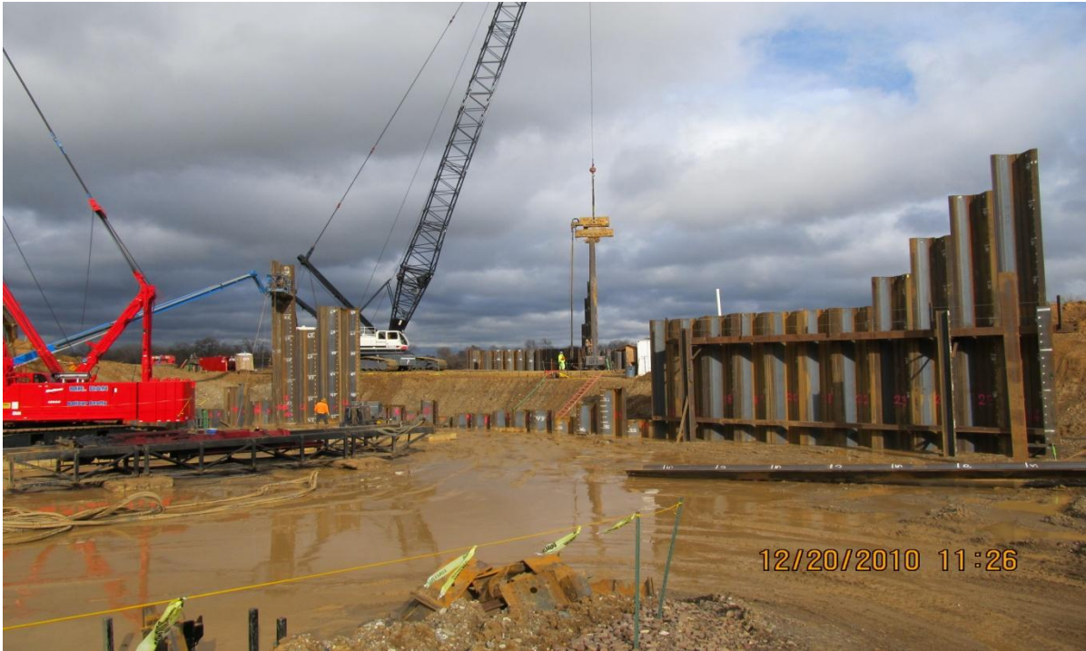
Balfour Beatty Pile Driving at the Forebay Fish Screen Area
