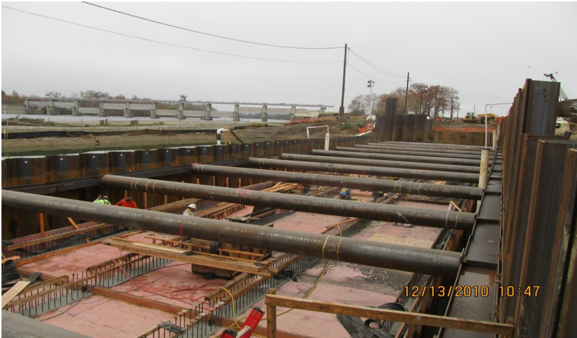
West Bay Builder's Siphon Barrel Structure Phase 1 Deck Forming
