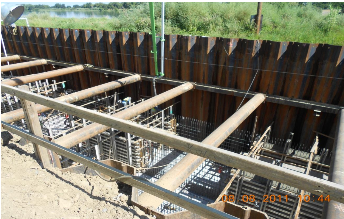
West Bay Builders performing wall placements.
