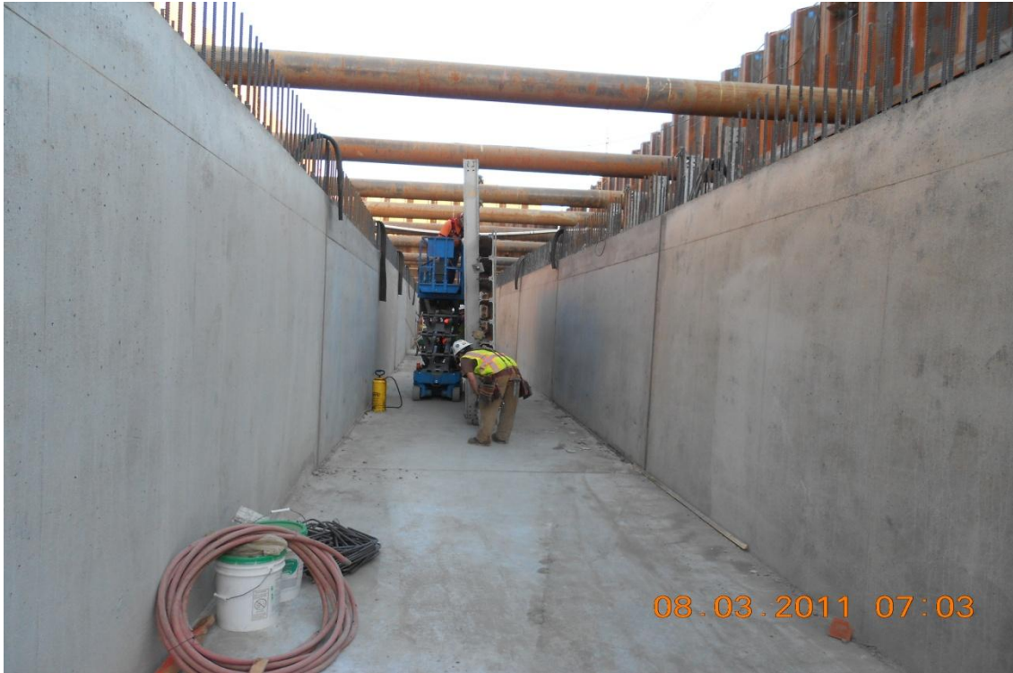
West Bay Builders crew moving wall forms to next bay.
