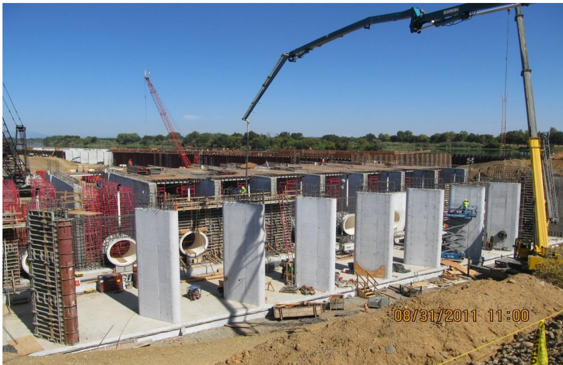
Balfour Beatty placing concrete on discharge wall with 2 pipe embeds.
