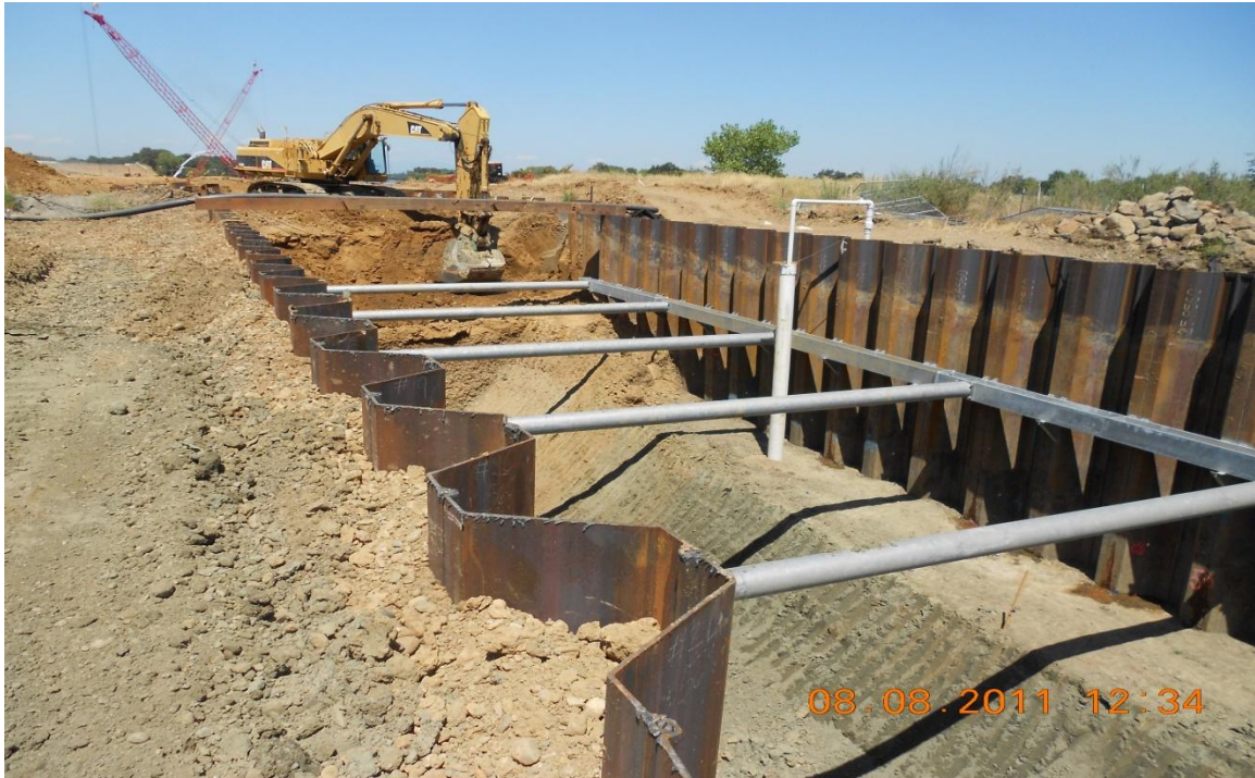
West Bay Builders subcontractor Meyers excavating ramp at upstream canal.
