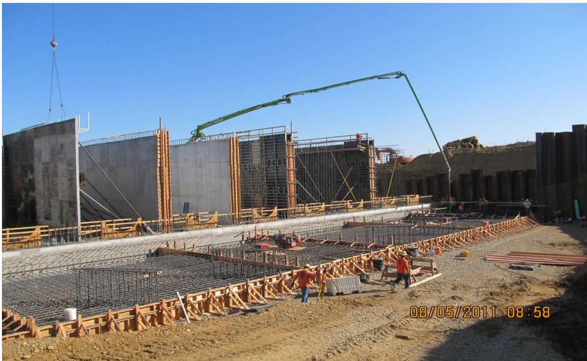
Balfour Beatty placing concrete in 4 afterbay slabs.
