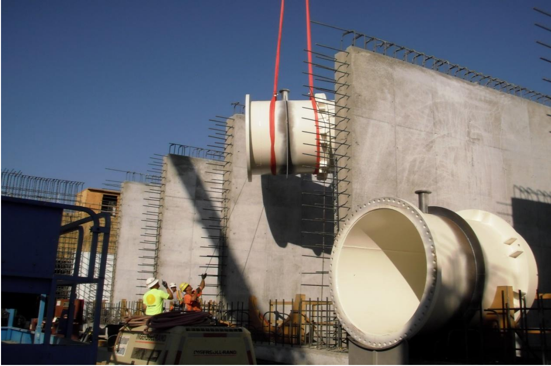
Balfour Beatty workers setting discharge pipe wall embeds into place.
