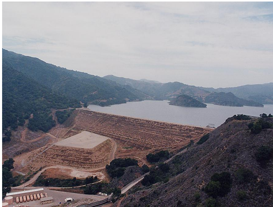
Casitas Dam and Reservoir
