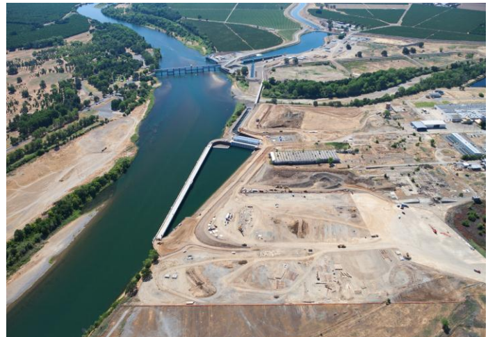
Red Bluff Pumping Plant and Fish Screen.
