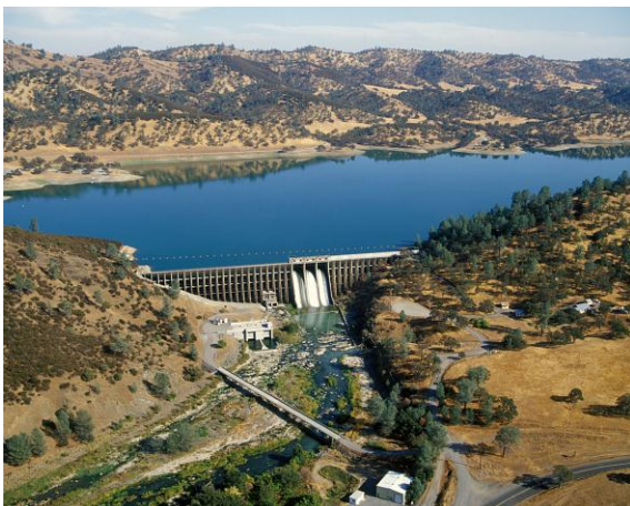
Stony Gorge Dam and Reservoir
