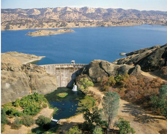
East Park Dam and Reservoir
