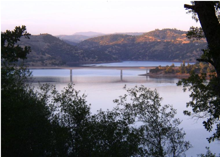
Stevenot Stanislaus River Bridge spanning New Melones Lake
