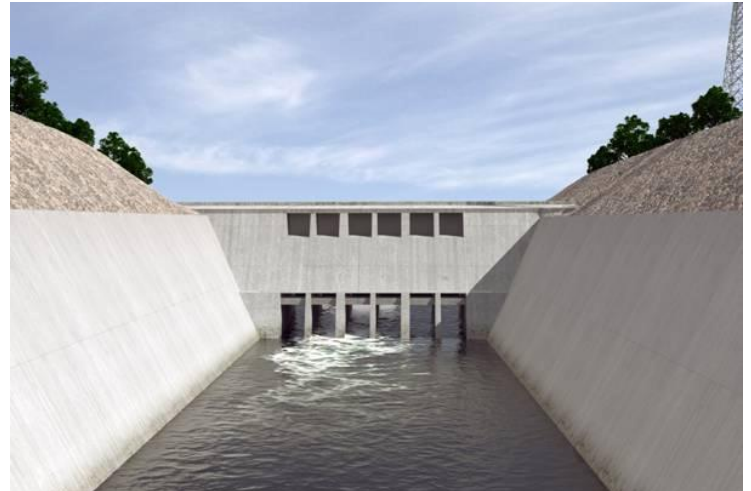
Artist's rendition of the completed auxiliary spillway gates.
