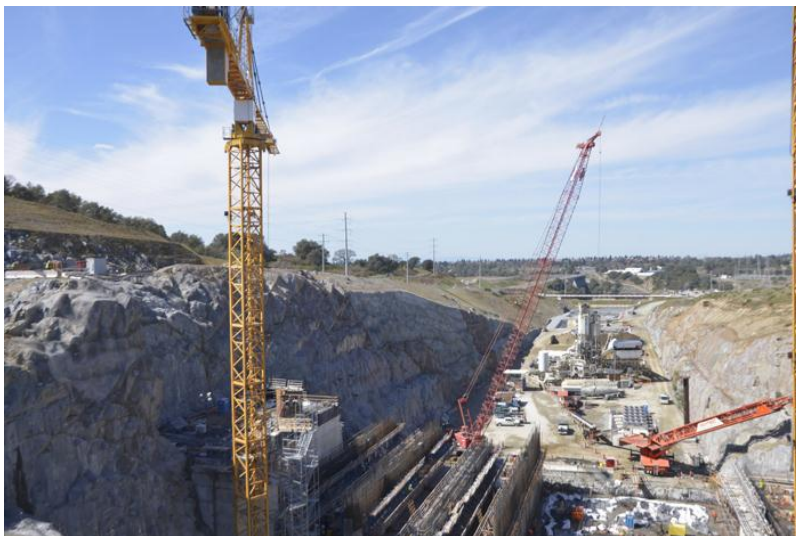
Construction of the new auxiliary spillway as of March 2013.
