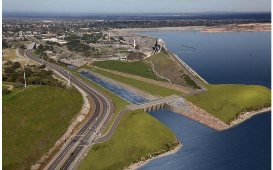
Artist's rendition of the completed auxiliary spillway.
