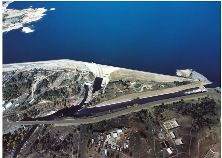
Artist's rendition of the completed auxiliary spillway.
