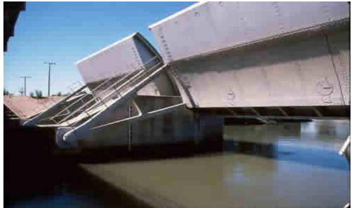
The Cross Channel gates in the raised position.
