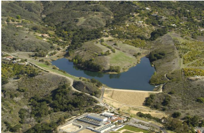
Lauro Dam and Reservoir
