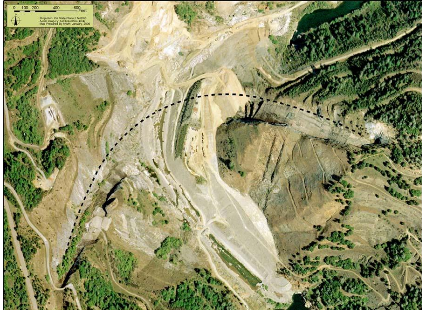
Aerial view of Auburn Dam site and foundation.
