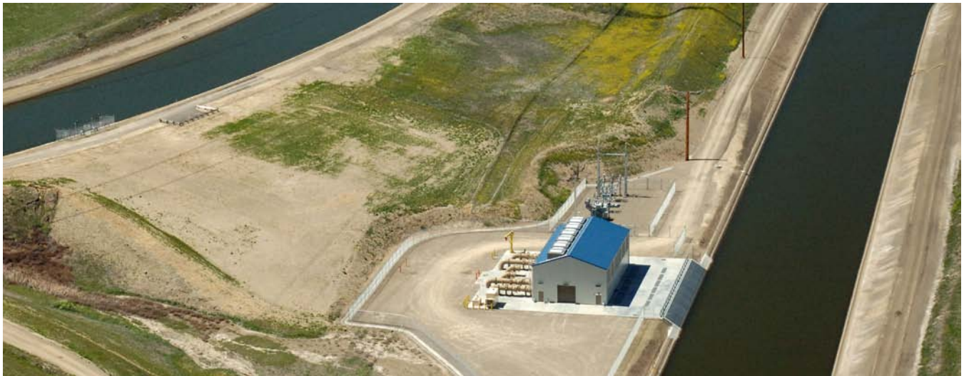
Intertie Pump Station located between the California Aqueduct and the Delta-Mendota Canals.
