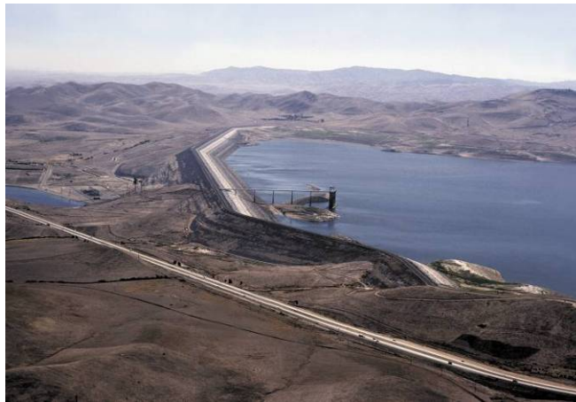
Figure 2-1. San Luis Reservoir
