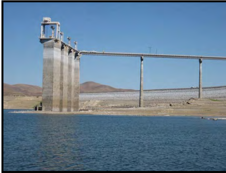
Figure 4. Outlet works intake towers and access bridge
