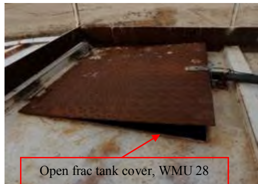
Olympus Stylus 8000, Photo #75; View of top of the leachate collection frac tank (Frac Tank 3) at WMU 28. Note the open cover.
