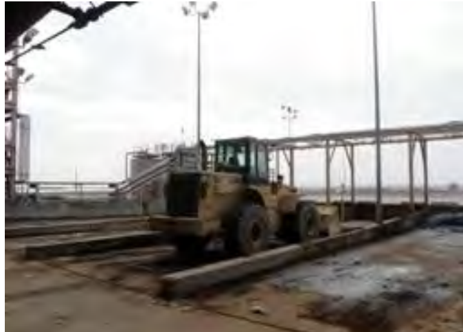
Olympus Stylus 8000, Photo #5; View of the bulk unloading bays at the STU, facing southeast.
