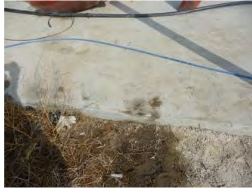
Panasonic Lumix DMC-TZ5, Photo #28; WMU 34; F039 leachate dripping on the ground.
