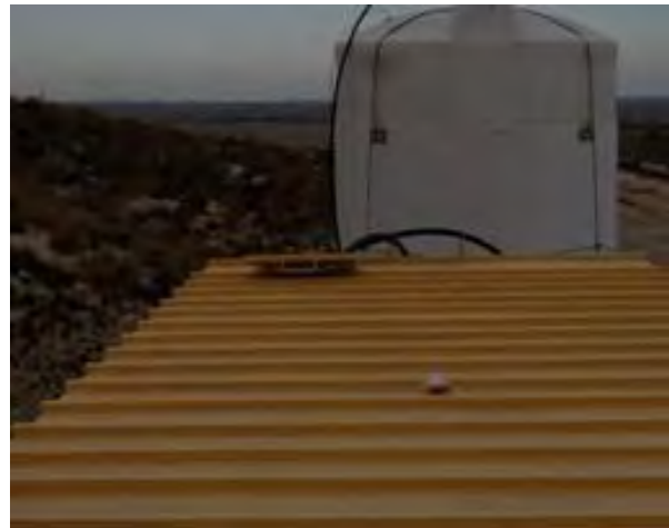
Olympus Stylus 8000, Photo #98; View of the leachate collection frac tank (Tank 80) at WMU 35, Cell #1, shown in Photo 96. Note the top of the container is open.
