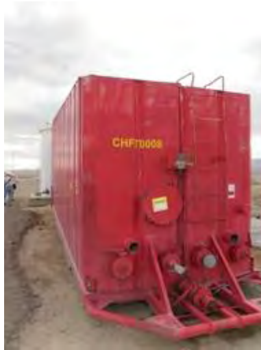
Olympus Stylus 8000, Photo #105; View of the red, leachate collection frac tank at WMU 35, Cell #3.
