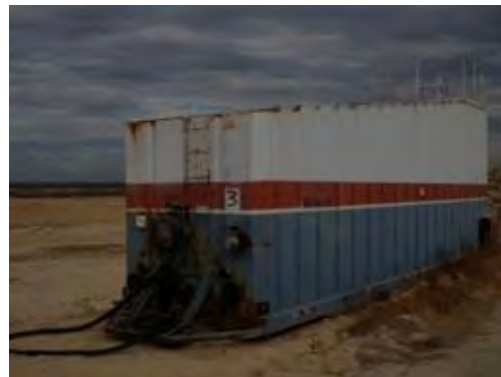
Olympus Stylus 8000, Photo #73; View of the leachate collection frac tank (Frac Tank 3) at WMU 28.
