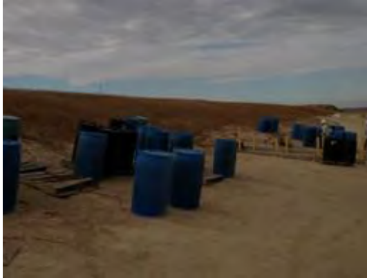
Olympus Stylus 8000, Photo #82; View of the leachate collection system and the less-than-90-day storage area at WMU 33, Cell #3.
