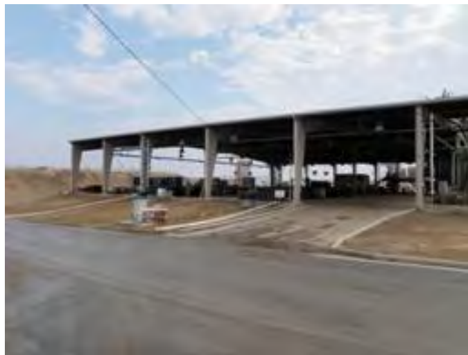
Olympus Stylus 8000, Photo #2; View of the drum storage area in the Stabilization/Treatment Unit (STU) area, facing northeast.
