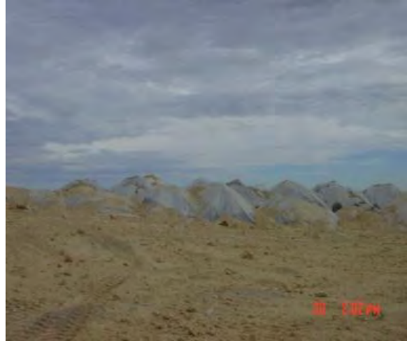
Sony Digital DSC-S75, Photo #13; View of the treated waste staging piles atop WMU 34 (under plastic tarping). View is from the southwest corner of WMU 34 facing east.
