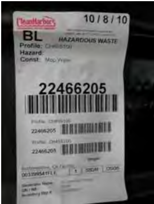
Olympus Stylus 8000, Photo # 12; Close-up view of a label with profile CH455100 (mop water) on a 55-gallon container in the drum storage area at DSHA Area 1. This waste is regulated as a California hazardous waste.
