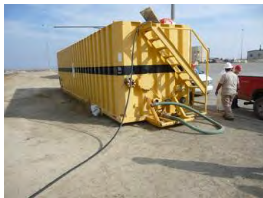
Panasonic Lumix DMC-TZ5, Photo #30; WMU 34 leachate collection frac tank, facing southeast.
