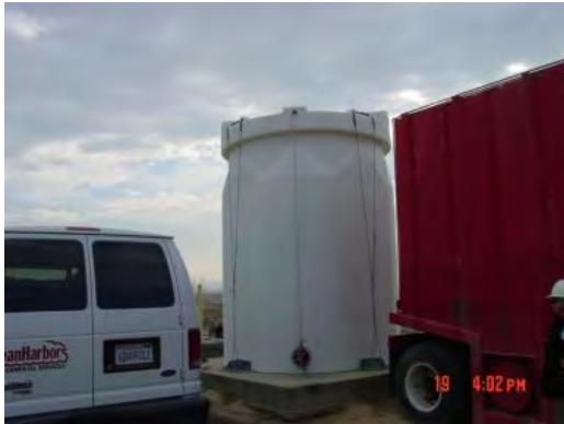
Sony DSC-S75, Photo #11; View of a 5,000-gallon, plastic, leachate collection tank at WMU 35, Cell #3, facing west.
