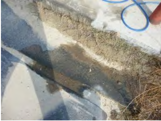
Panasonic Lumix DMC-TZ5, Photo #19; F039 leachate drippage observed on the ground at WMU 34.
