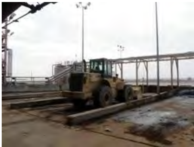
Olympus Stylus 8000, Photo #5; View of the bulk unloading bays at the STU, facing southeast.
