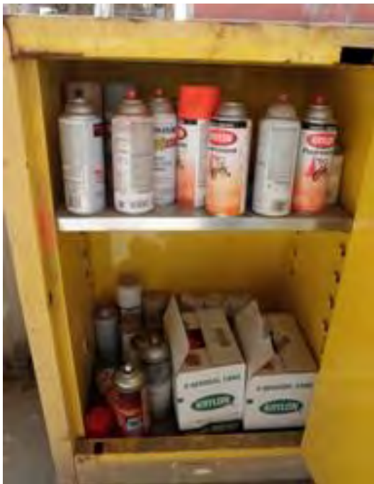
Olympus Stylus 8000, Photo #47; View of a flammable storage cabinet at the STU, holding aerosol products.
