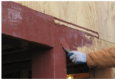
Installed with gun and putty knife or spreader
