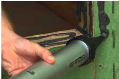
Installed with gun and putty knife or spreader
