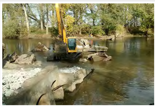
Backhoe removing last Eel River dam. Credit: Donovan Henry, USFWS
