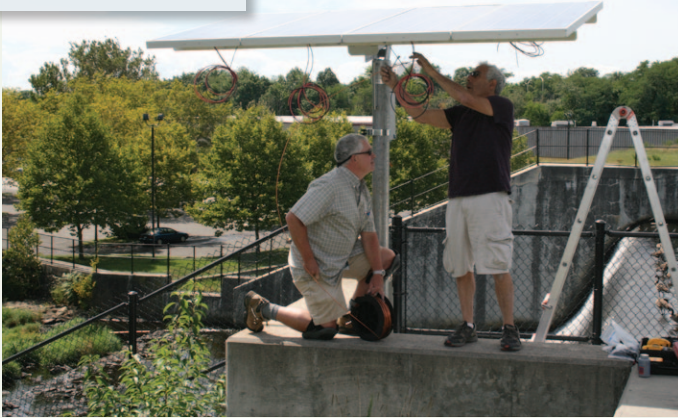
Installing solar panels at the fish ladder
