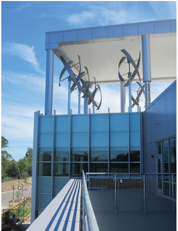
Wind turbines and green roofs at the LEED Gold-certified Fairchild Wheeler Inter-District Magnet High School, which offer a 21st century STEM (Science, Technology, Engineering and Math) project-based curriculum focusing on three areas: Information Technology, Biotechnology/Zoological science and Physical Science, Math and Aerospace/Hydrospace Engineering.
