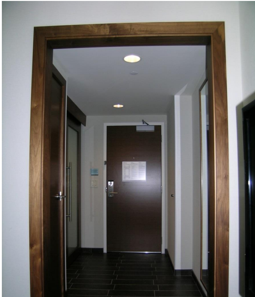
Figure 5: Guest room entry area, showing the positions of the two LED downlights. (PNNL photo – flash photography was used; the photo does not accurately portray the lighting effect.)
