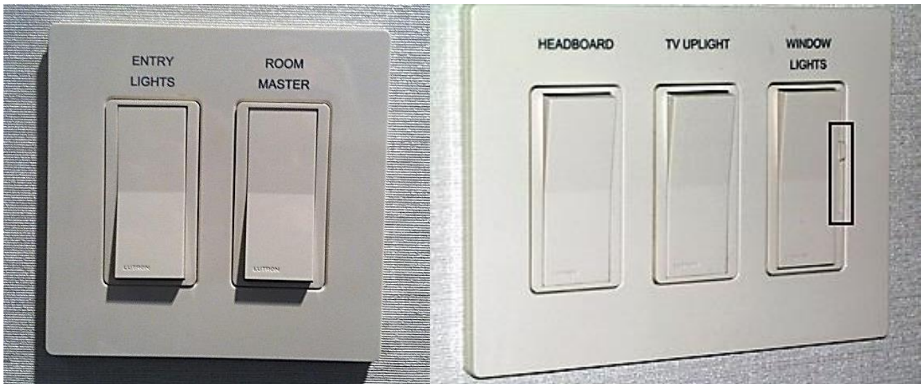
Figure 11: Entry area (left) and bedroom (right) switches with slide dimmer (outlined) for window lights (PNNL photo)
