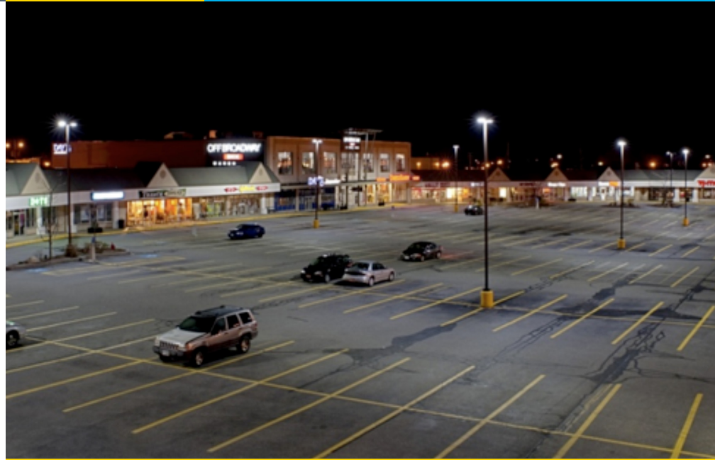
Parking lot after installation of LED luminaires
