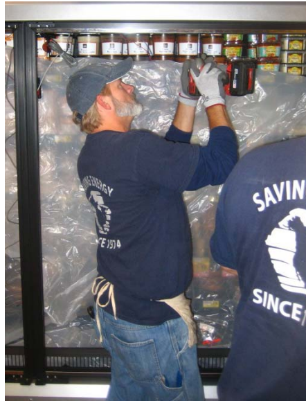
Figure 4: Installation of door frames
