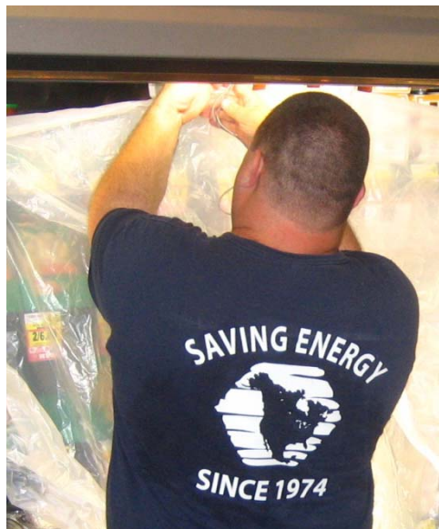
Figure 5: Wiring of new lighting fixtures
