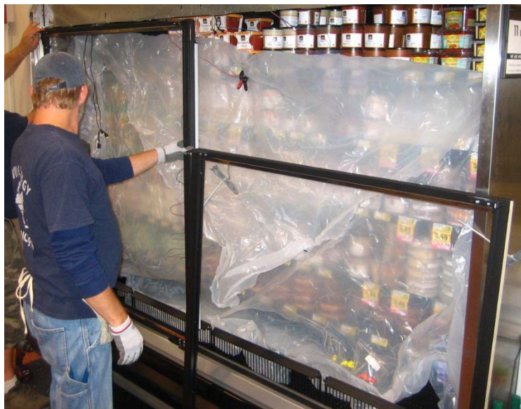
Figure 3: Fitting and placement of door frames
