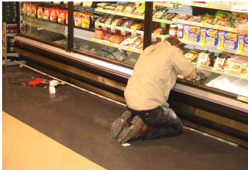
Figure 9: Expansion valve adjustment
