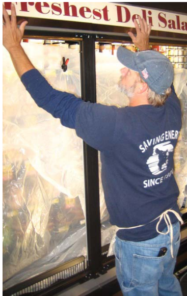
Figure 6: Replacement of top canopy
