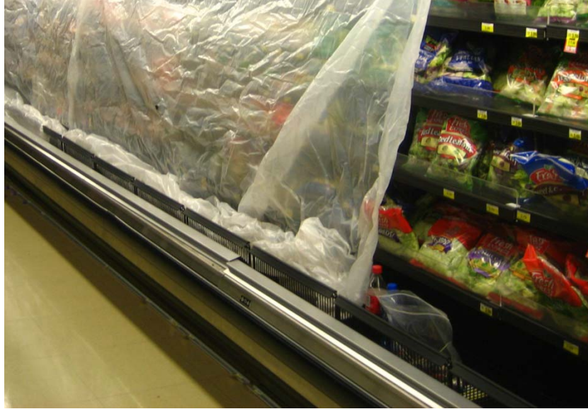
Figure 2: Covering of product and layout of new bottom rail
