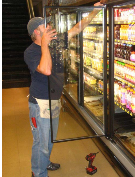
Figure 8: Hanging the doors
