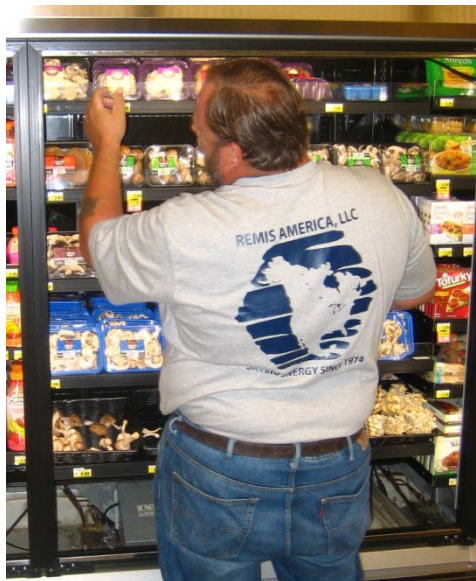
Figure 7: Gasket installation
