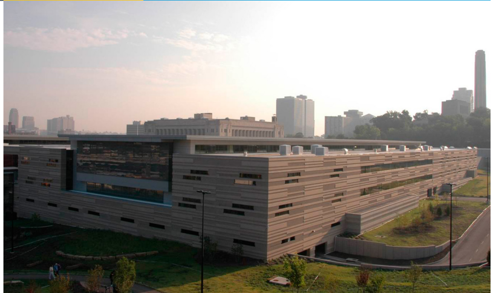
MC Realty Group, LLC, replaced 1,500 old metal halide fixtures in a five-story parking garage in Kansas City used by federal employees of the Internal Revenue Service. MC Realty achieved a 76% reduction in energy use by replacing the metal halide fixtures with T8 linear fluorescent fixtures. Installing motion sensors on two-thirds of the fixtures accounted for 22% of the savings.
