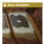
NOTICE: If air sealant is a foam plastic, it must be covered with an approved thermal barrier (e.g. rockwool, slag wool).
