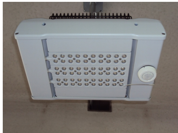
Figure 2.9. Close-up of LED luminaire and integral motion sensor (metering light pipe also shown)
