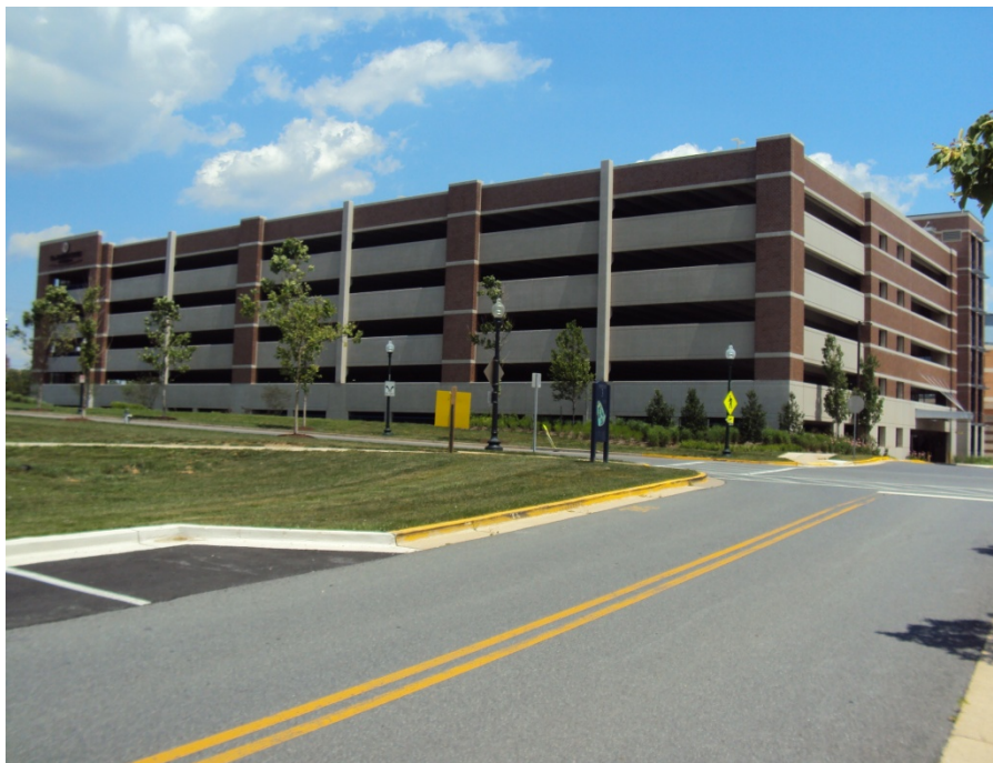
Figure 2.6. Site of exterior parking structure GATEWAY demonstration
