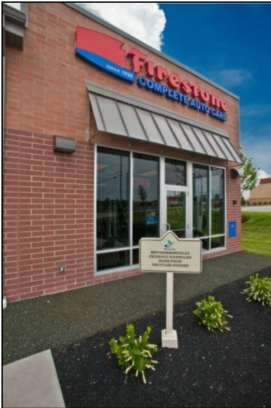
Firestone Complete Auto Care Smyrna, Tenn. Gold LEED Certified
