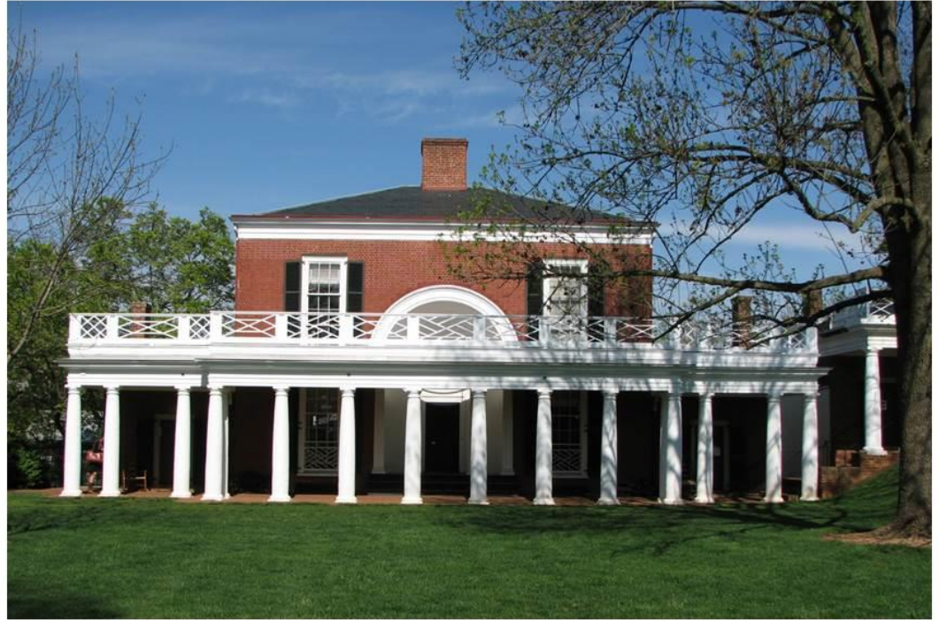
Pavilion IX Renovation
