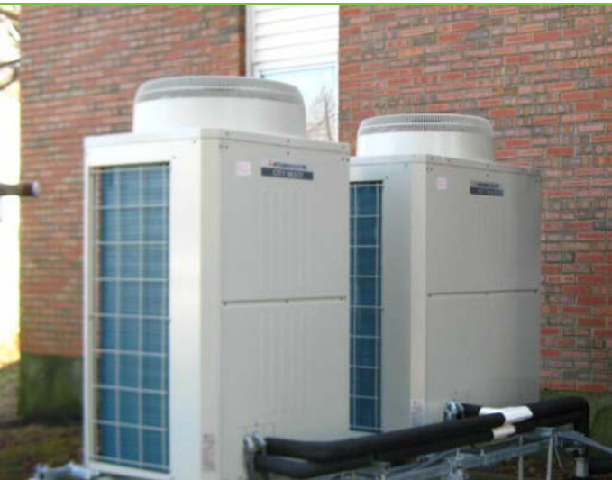
Winthrop Public Housing: Outdoor Condenser Unit for Heat Pumps
