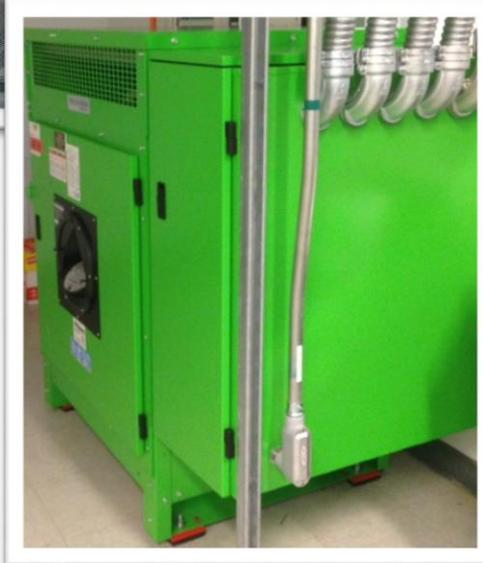
Typical Performance Data: High Voltage—15 kV Class; Low Voltage—600 V Class
