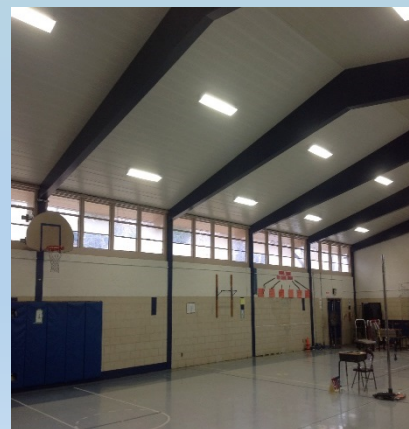
Gym Lights After Retrofit
