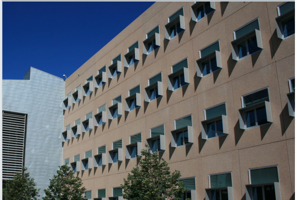
NREL Research Support Facility, photo credit: Bill Gillies, NREL
